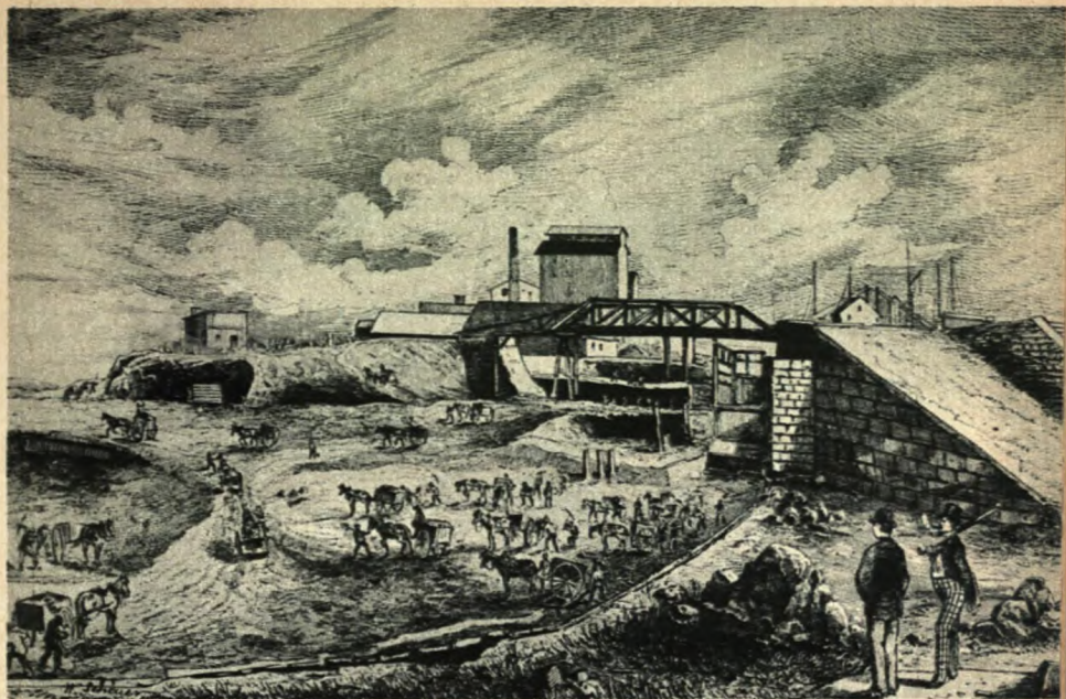
Early excavation operations on the old Lachine Canal connecting the Port of Montreal and Lake St. Louis
