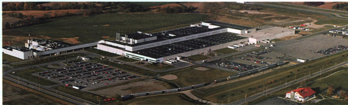
Toyota's plant in Cambridge, Ontario
