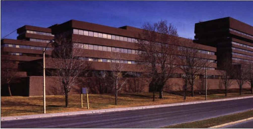
Canada's Department of Foreign Affairs and International Trade (DFAIT) had traditionally relied on a secure telex system to link its Ottawa headquarters and its 146 embassies, consulates and missions around the world.
