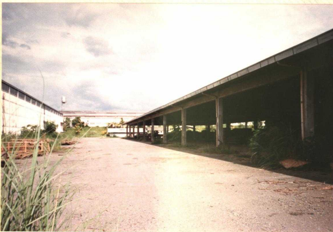
No. 4. Lumber shed on right. Woodworking Plant in background. Note reinforced concrete shed construction and blacktop paving throughout.
