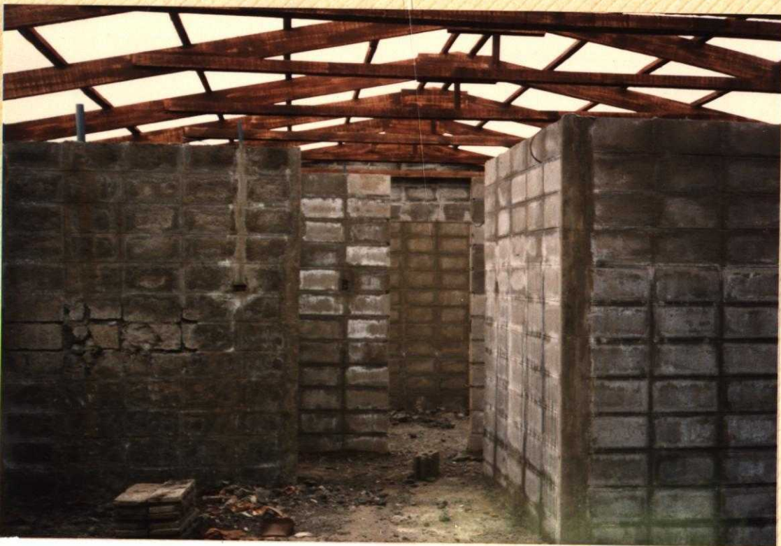
No. 63. Interior partitions entirely of hollow block. Bathroom enclosure on right.
