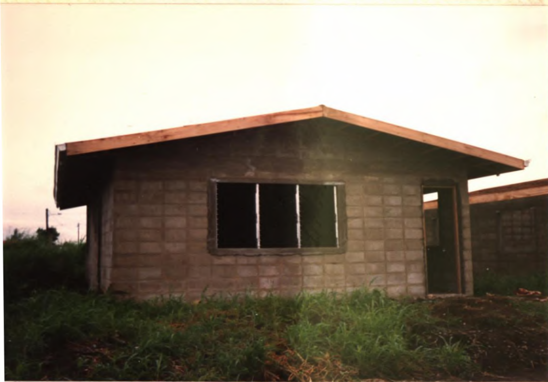
No. 67. Door and window frames installed and corrugated sheet metal roof and gutters complete.
