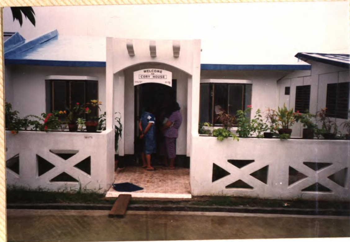
No. 36. "Cory House" front entrance.
