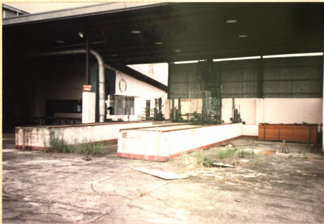
No. 8. Sawmill log deck and headrig. Note full concrete yard paving and steel building construction.
