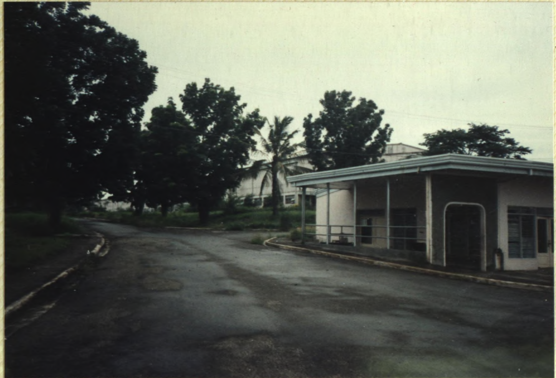
No. 1. Entrance to NHC Complex. Guardhouse and employee time clock station in right foreground. Woodworking plant in background.
