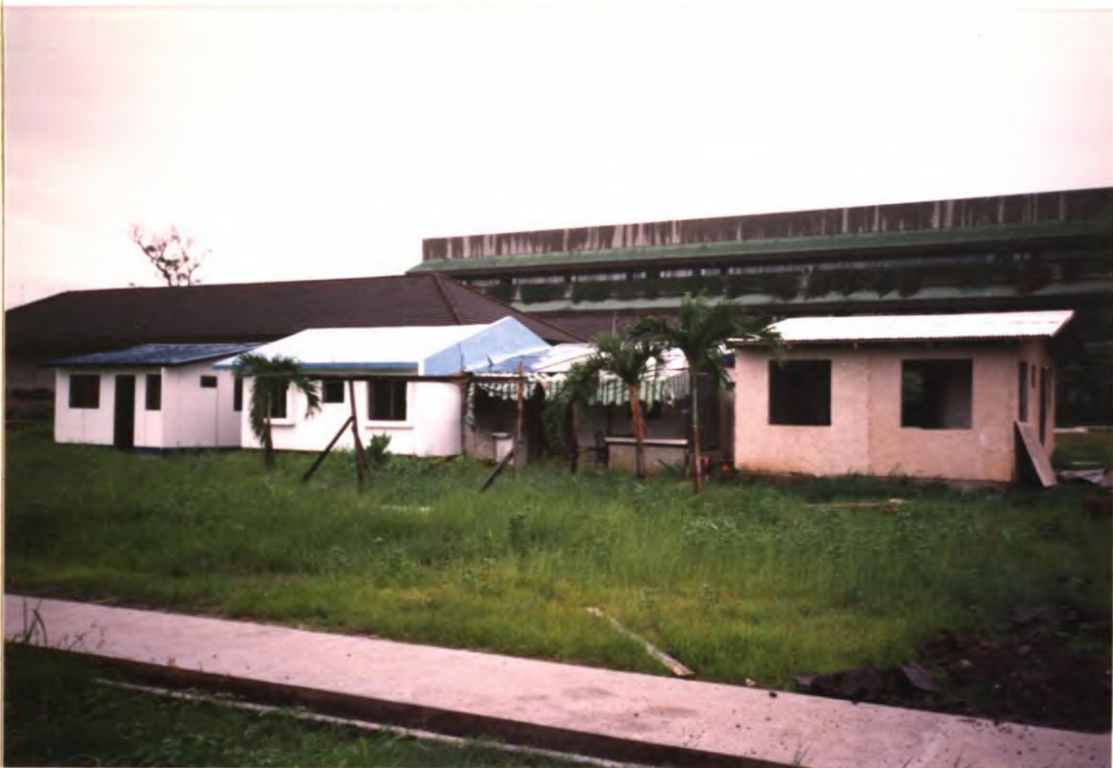
NO. 29. FOUR DISPLAY HOMES IN NHA COMPOUND.
