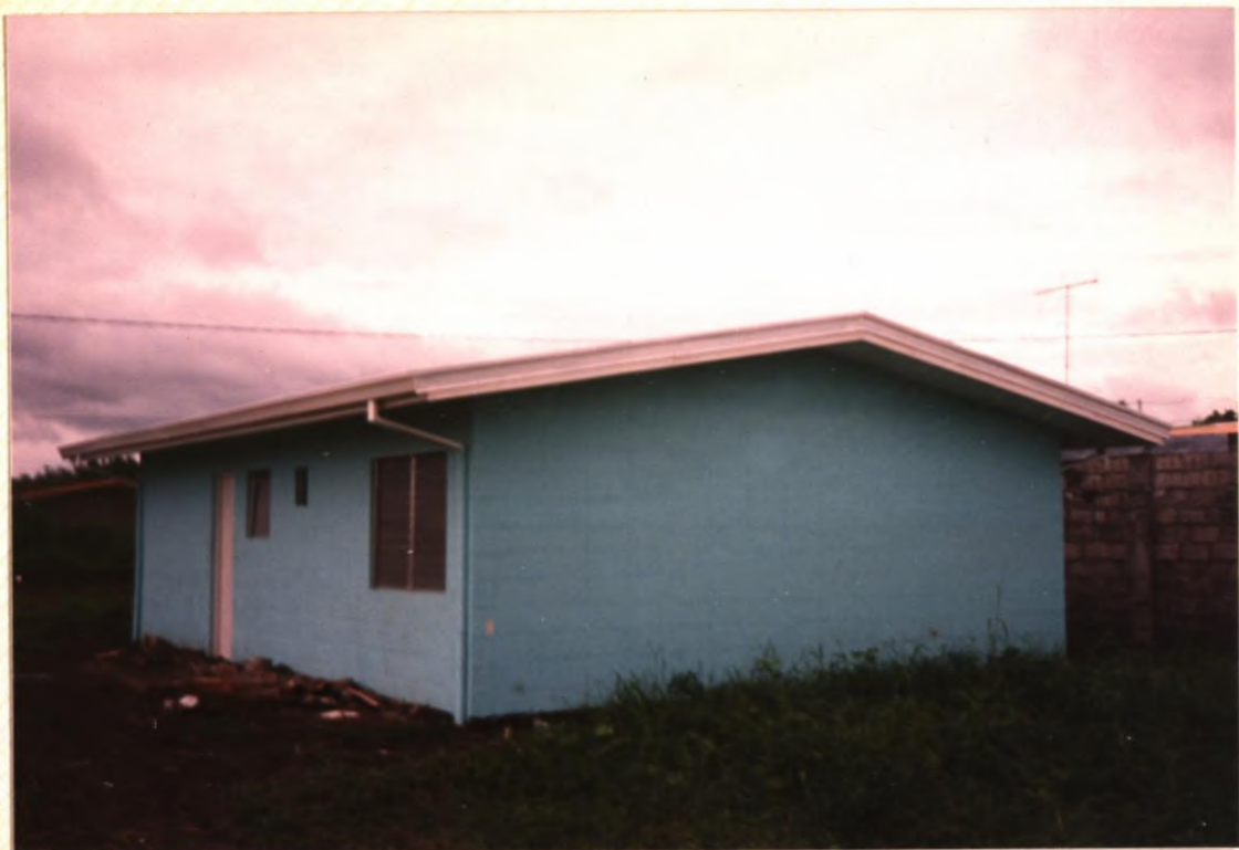
No. 69. Completed house, including exterior and interior finishing.
