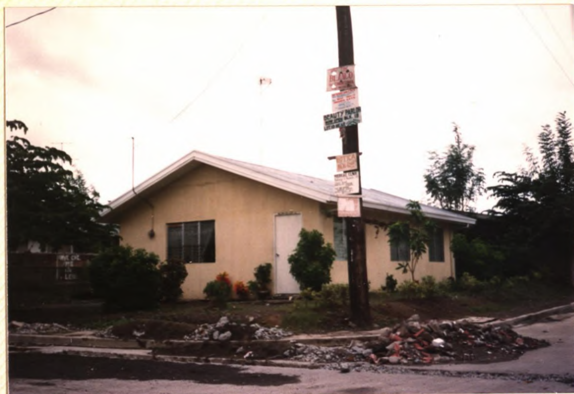
No. 73. A finished house built via the pre-cast panel method before this system of construction was abandoned in favour of the hollow block style.
