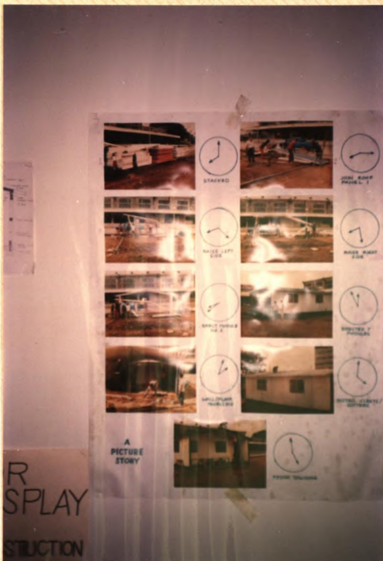
No. 35. Poster on Lukut House showing stages of complete on-site assembly in one day.
