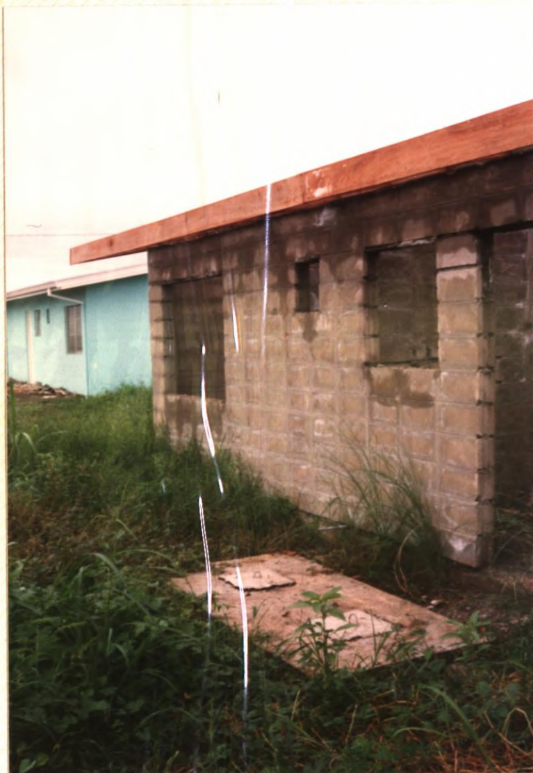
No. 65. Septic tank installed at ground level.
