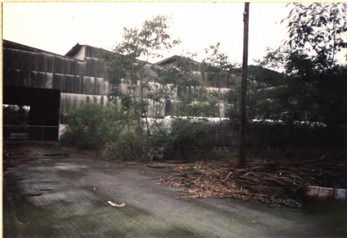
No. 24. Outside view of lightweight concrete plant building.
