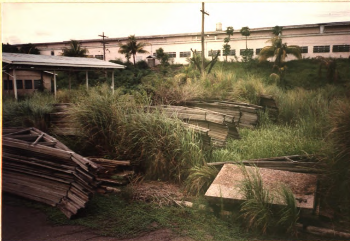
No. 27. Pressure treated, pre-fabricated gangnail roof trusses left in the yard.
