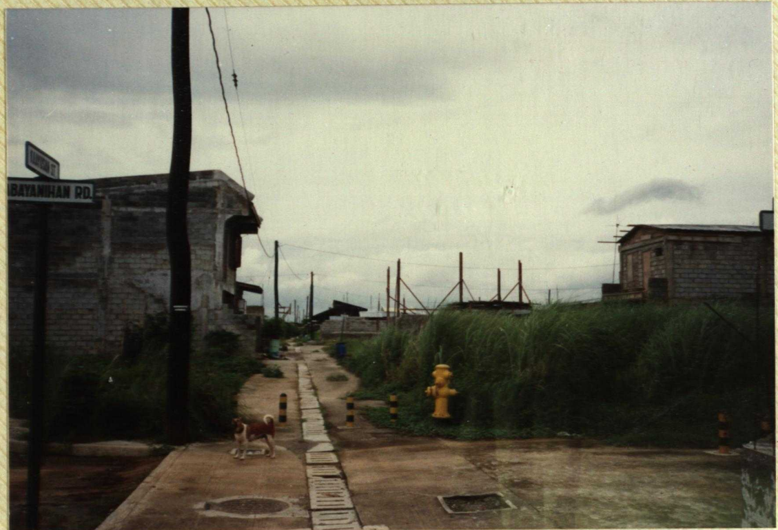
No. 57. Partially completed homes. Owners have purchased a lot and are building as they have funds available.
