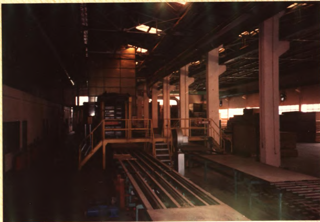
No. 18. OSB Press line with 5-opening, 4x16 ft. press in background.
