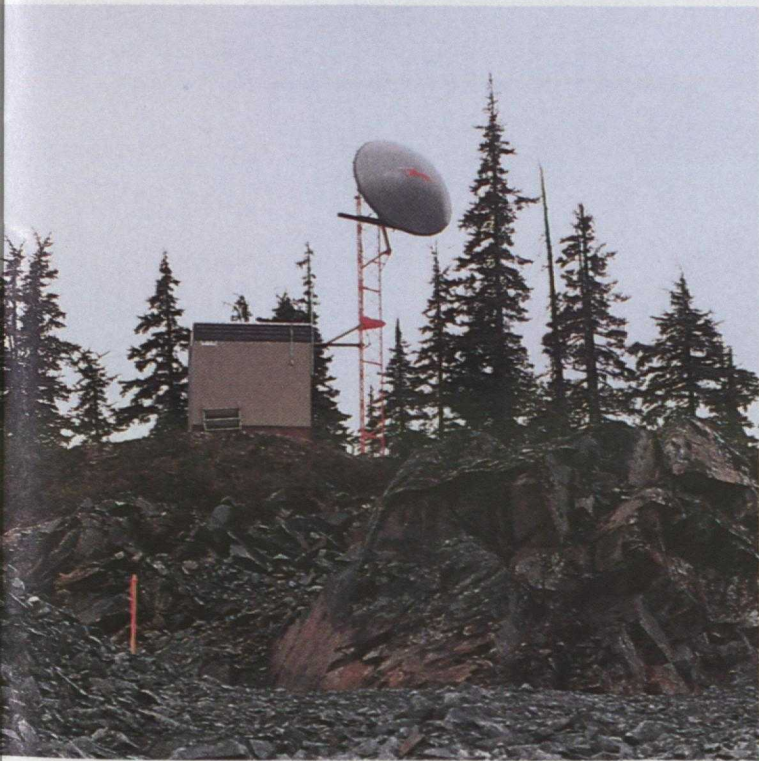
■ Typical rural microwave radio communications installation — Westmin Mine site, Stewart, B.C.
