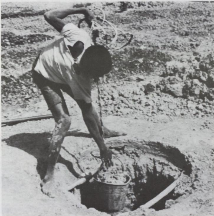
*The manual excavation of a well in Niger.*
