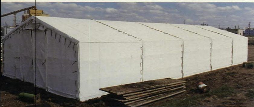
Shelter shown in photo, with outside and inside view, has 12 m x 30 m x 3.6 m eave with peak height of 6 m. Note that the translucent fabric allows for day-time use without additional lighting required.
