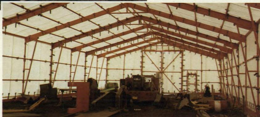
Norseman Shelters manufactures portable buildings made with a steel frame and fabric cover and designed for fast, easy erection by unskilled personnel. Norseman's pin and pocket assembly system requires no bolts, allows personnel to keep their gloves on, and eliminates the need for special tools. The frame and fabric dismantle into easy-
