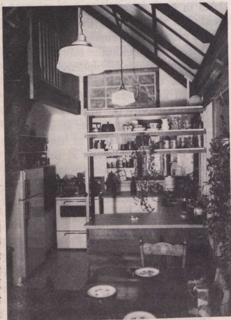
Dining and kitchen view with Trombè wall vents open on upper right. Solar water collectors are above cathedral ceiling.
