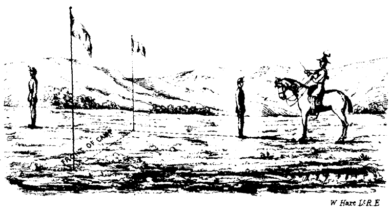
3 LAYING OUT A RIGHT ANGLE. First Method.
