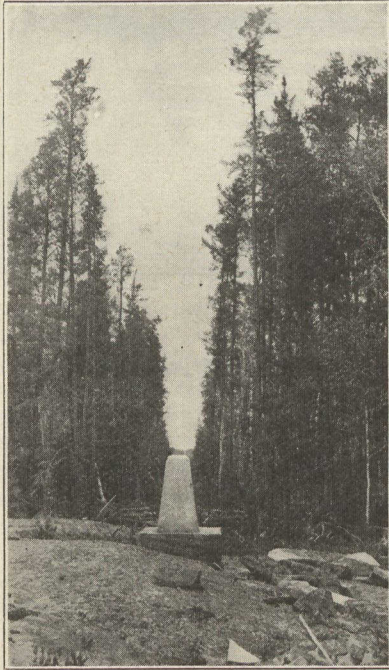
Manitoba - Ontario boundary — This picture shows how the boundary has been marked by a cleared line through the forest and by concrete monuments. An idea is also given of the character of the timber.
