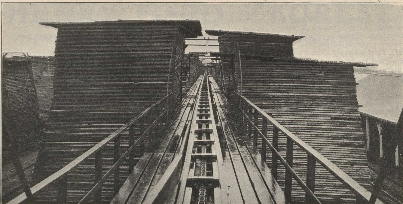
The chain conveyor which carries the lumber from the mill to the lumber piles in the yard. Thus saving man and team handling. From the yard the lumber goes to the body plant, where it is made into parts for the Ford car.
