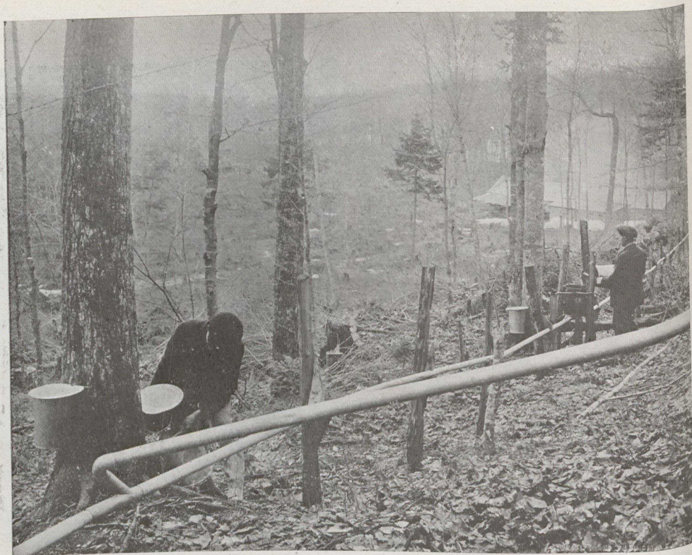
Employing pipe lines to carry the maple sap to the evaporator.
