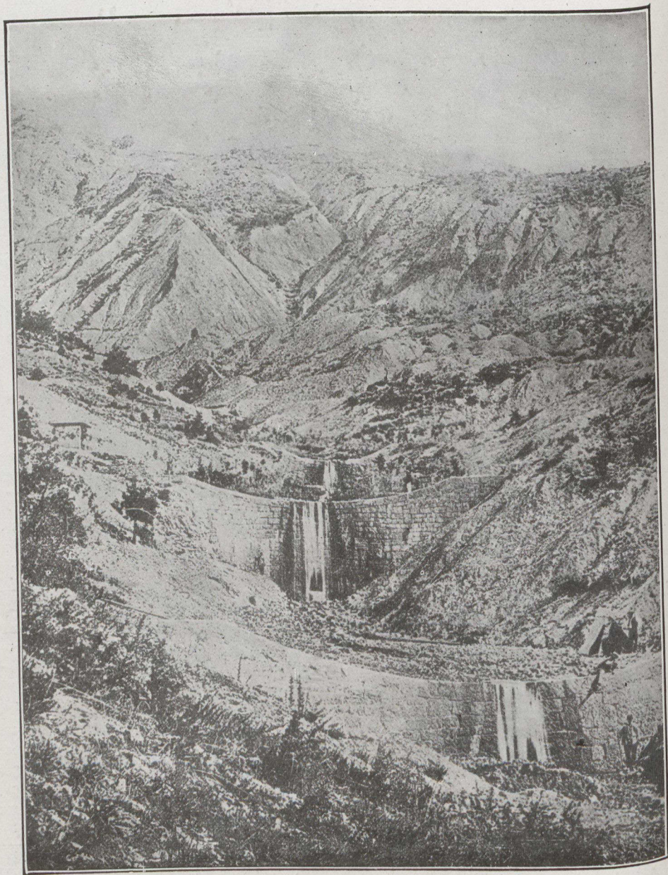
These pictures graphically illustrate the success of torrent control in France. The first shows a torrent in the Lower Alps, the bed of which has been built up by barrages behind which sediment collects. This photograph was taken in 1887; note what has happened since, as shown on opposite page.
