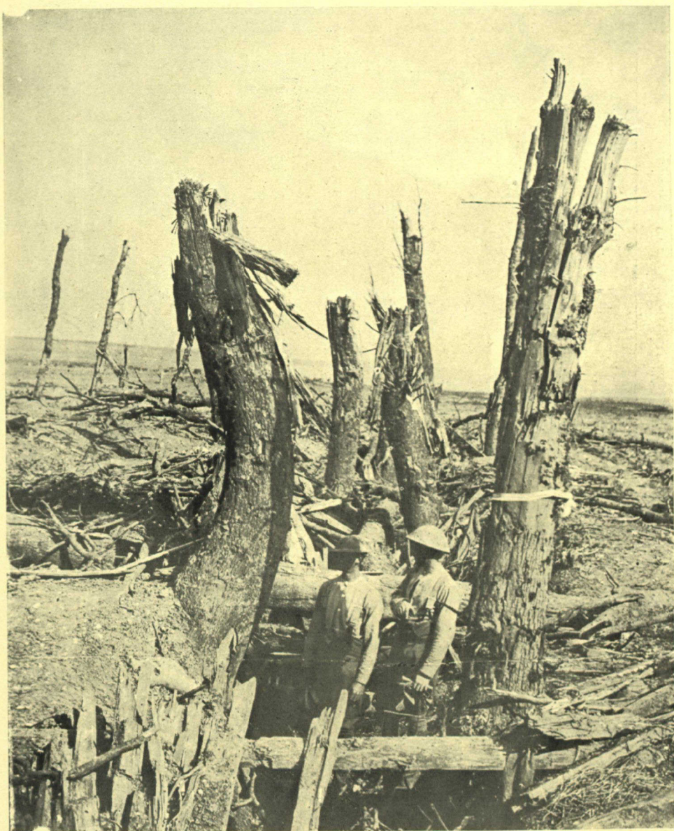
Utilizing the smashed trunks of trees for trench protection.
