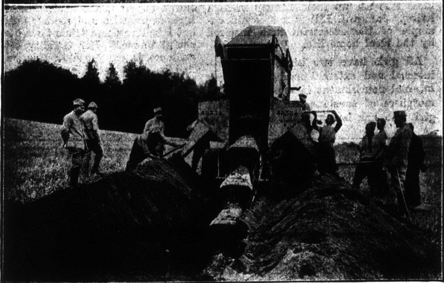
Upper—Side view of the powerful French tractor which builds trenches and constructs breastworks as it travels along. The photo gives an intimate view of some of the mechanism which does the work and shows French soldiers operating the machine. Lower—Rear view of the tractor, showing huge scoops which remove dirt, and other parts of the mechanism which does the work of scores of men.
