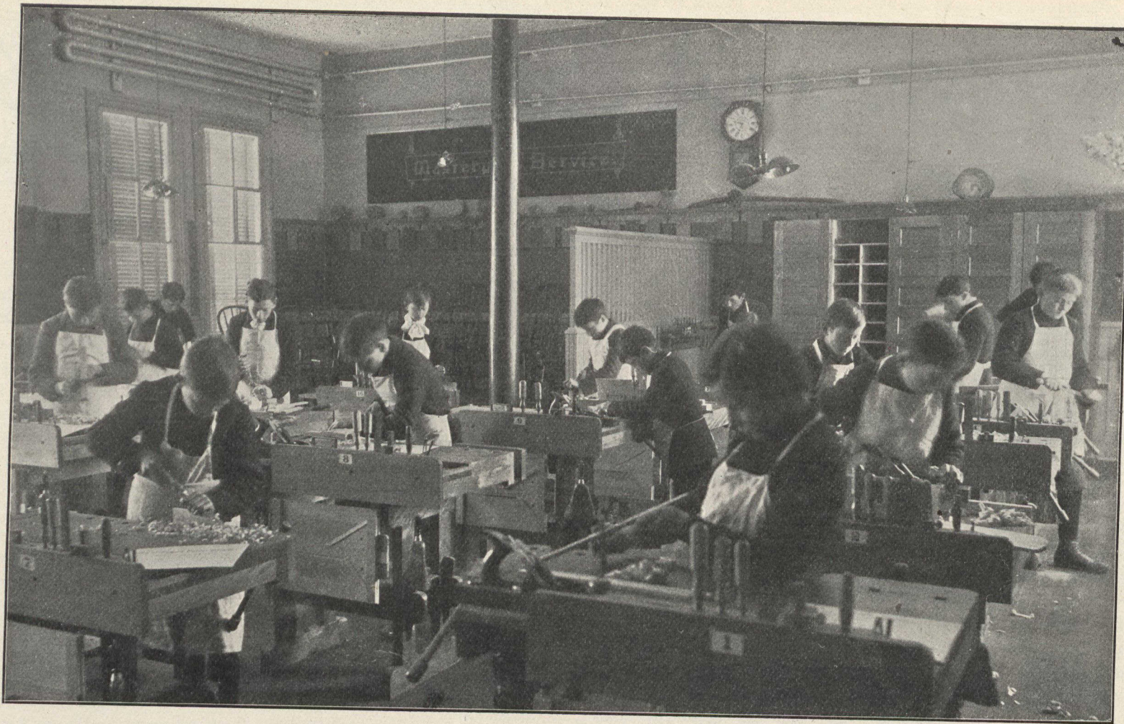
Manual Training Room, Creighton Street Public School, Ottawa.
