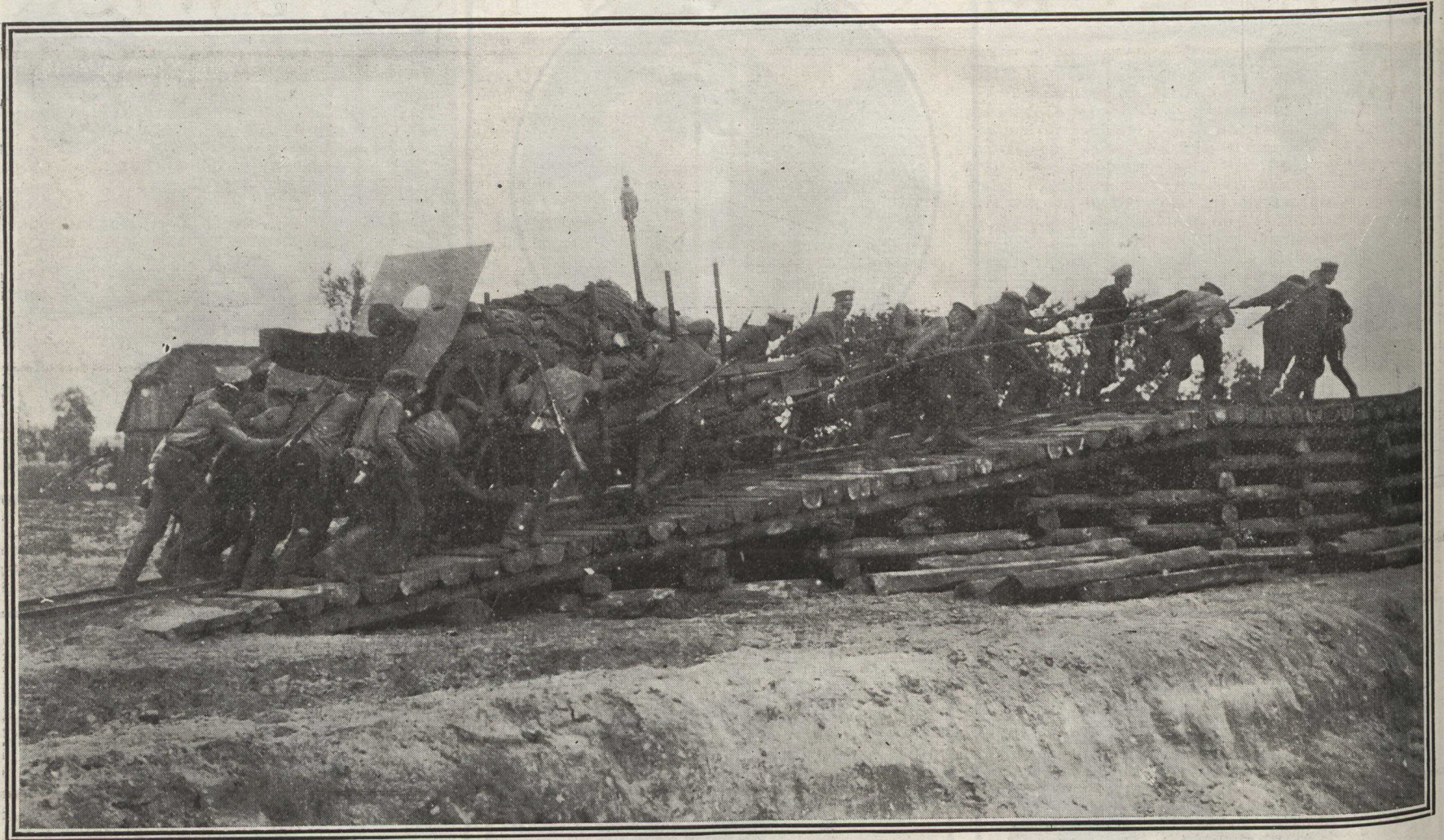
A great painter might have made this picture, which as an epic rivals any of the fabulous labours of Hercules. These Russian sappers and gunners are hauling a heavy field cannon over a specially built track on to a temporary platform built of tree-trunks and pine-wood slabs. The gun is mounted on two sets of wheels, big wheels running on the ground, low truck wheels operating on railway tracks. It was not built for gasoline traction, and is not a siege gun. It is a field-piece capable of transportation anywhere, even over the swamps of Russia. The only problem seems to be getting men enough around the gun to move it. And this picture of moving a great Russian gun, taken in Poland, is one of the great epical photographs of the war.
