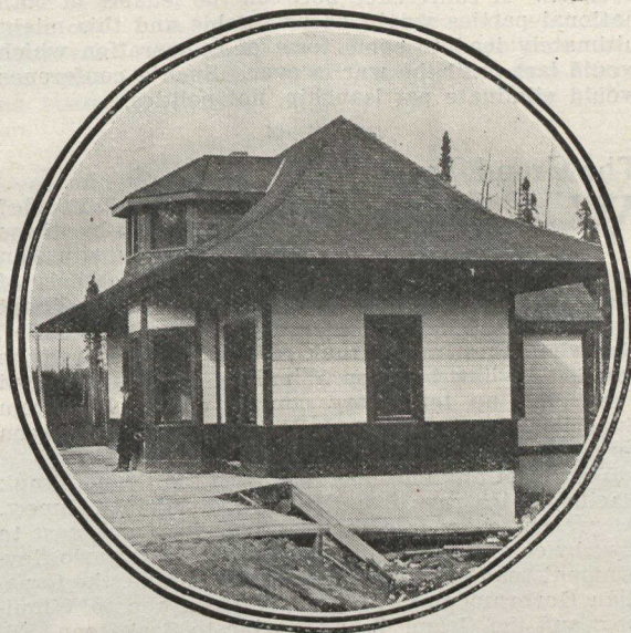
The type of station building used along the N.T.R.
