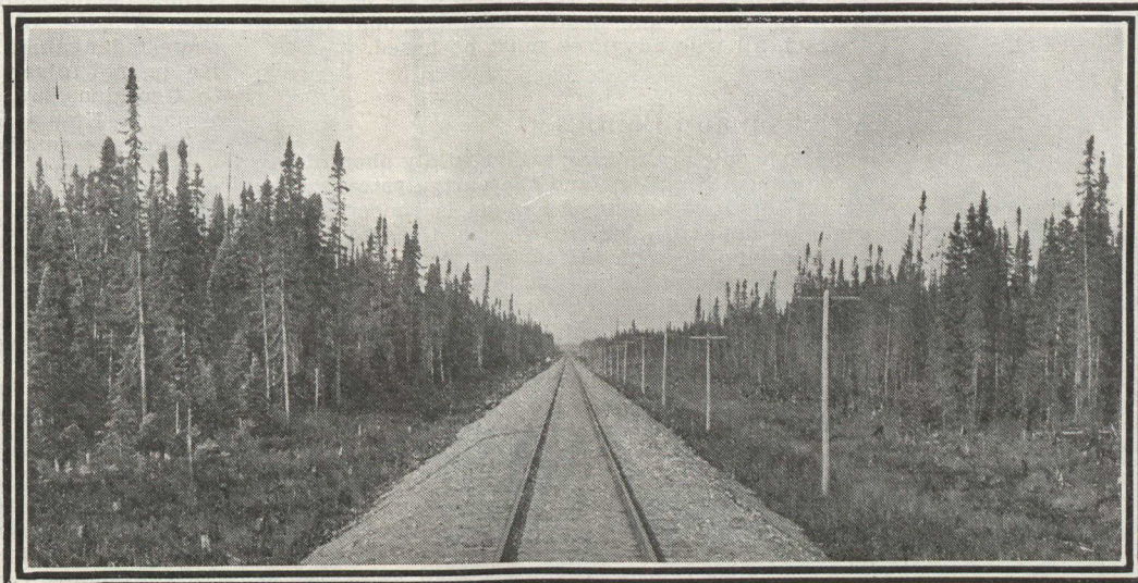
With low grades and easy curves, the new National Transcontinental runs from Quebec to Winnipeg, a distance of 1,350 miles.
