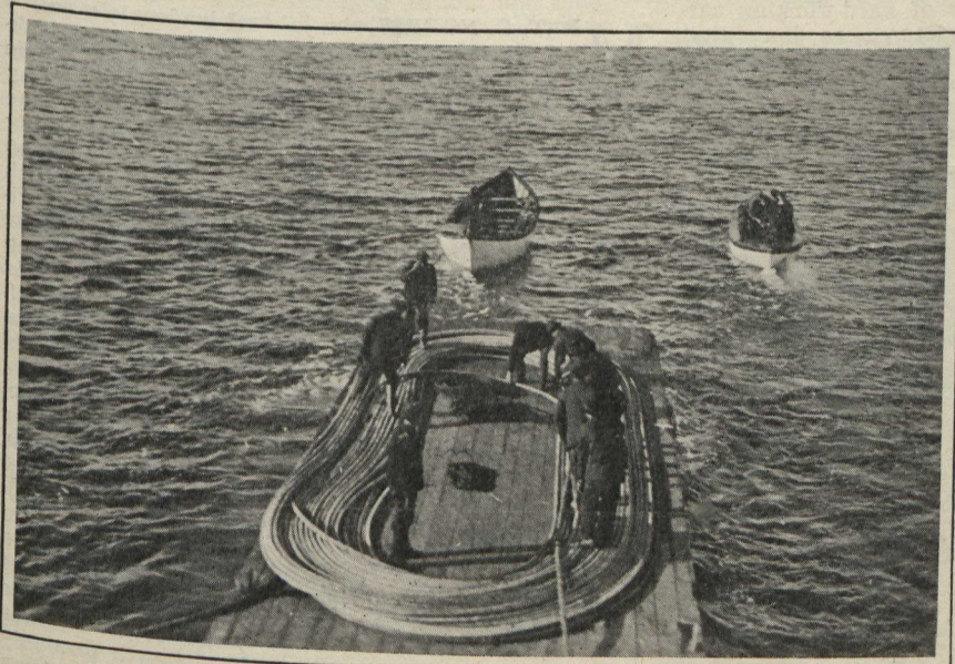
These two photographs illustrate the fairly easy task of laying a cable from Caribou, Nova Scotia, to a point near Charlottetown, P.E.I. It will be used entirely for telephone communication, and the first conversation over it was between Premier Borden and Premier Mathieson.
