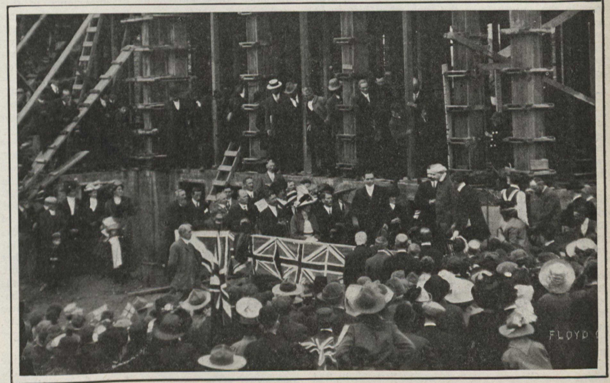
Sir Richard McBride laying the Corner-Stone of the new $50,000 school in Chilliwack, B.C. A feature of the event was the massing of the school children of the Valley to see the ceremony.
