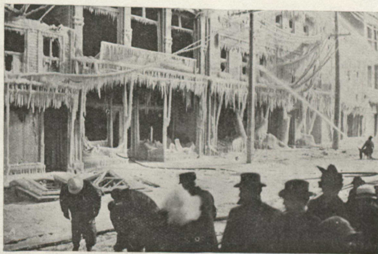
After the fire on Barrington Street.
