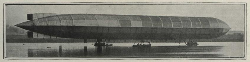
At daybreak a few mornings ago this monster airship was successfully launched at Barrow, England. The mighty aerial cruiser is 512 feet long and has an external diameter of 48 feet. It is made of duralumin, an alloy as hard as steel and only one-third the weight. Its seventeen gas bags are inflated with hydrogen and are capable of lifting 21 tons. It is controlled by horizontal rudders forward and aft on each side, with vertical rudders aft above and below the stern. Photographs by Topical.
