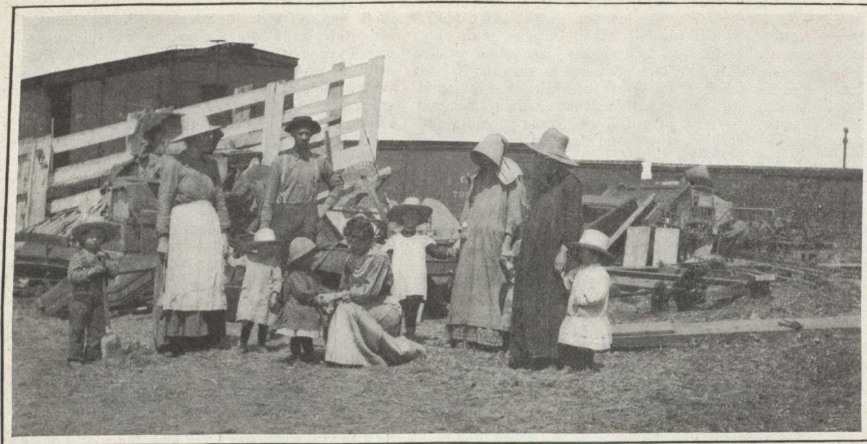
AT THE END OF THE STEEL WHERE THE TRAIL BEGINS
