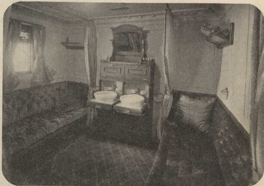
A State-Room on the Bridge Deck
