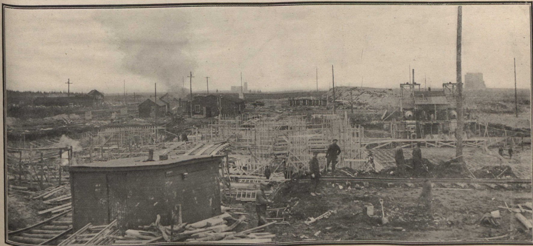
Canada, has now the largest Wheat Elevator in the world, the C.N.R. Elevator at Port Arthur with a capacity of seven million bushels. Here is shown the foundations for the first unit of the Grand Trunk Pacific Railway Elevator, planned to an ultimate capacity of forty million bushels. This is being built on "The Mission," across the Kaministiquia River from Fort William, the terminus of the Lake Superior Branch of the G.T.P. It was hoped this Elevator would be ready for the shipping season of 1909, but this is doubtful. In the distance, beyond the River, tower some of the present Elevators of Fort William; these are six or seven in number and have a present capacity of twenty million bushels.
