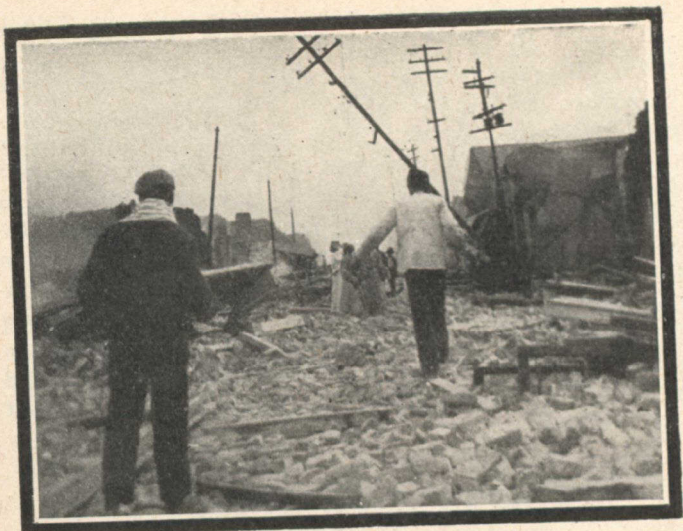
Harbour Street, looking East. Much damage was done in this section.
