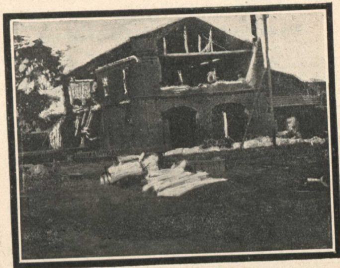
A Building wrecked by the Earthquake.
