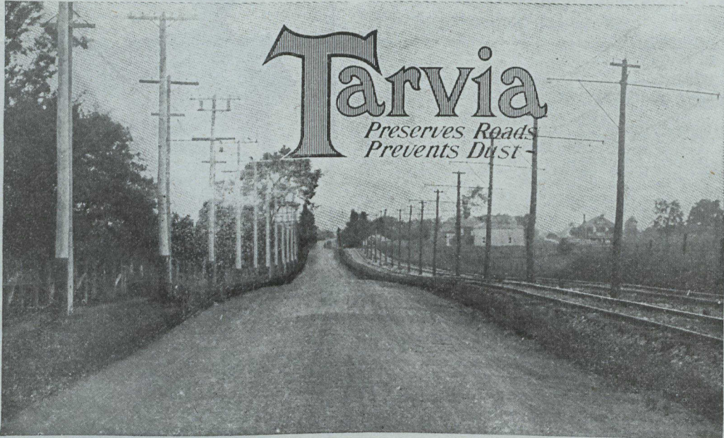
Galt-Preston Road, Waterloo County, Ontario, Treated with "Tarvia-B" in 1914 and 1917
