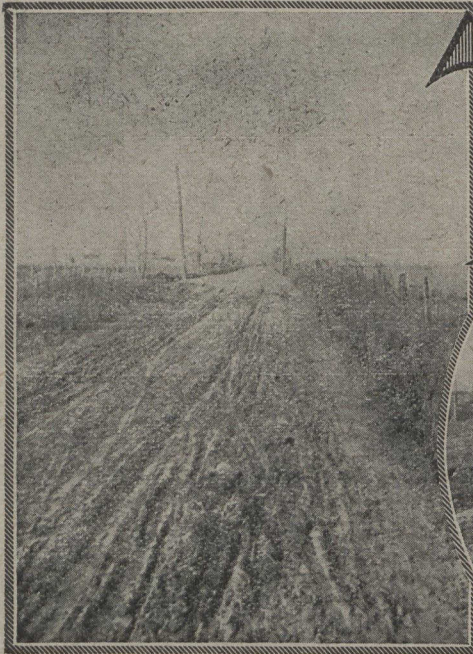
Beaconsfield Station Road, Beaconsfield, P. Q. This is what happened when the road was weaker than the automobile.
