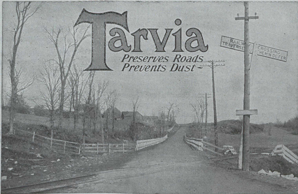
Sherbrooke-Derby Line Highway, (Provincial Government) Near Lennoxville, Quebec 7 miles of Tarvia Filled Macadam (Slag)
