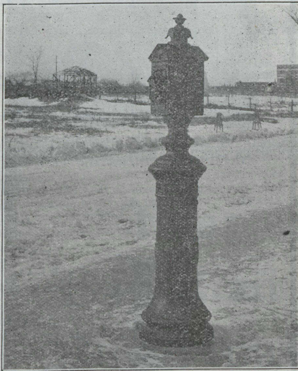
Fire Alarm Box Mounted on Street Pedestal, Outremont, P.Q.
