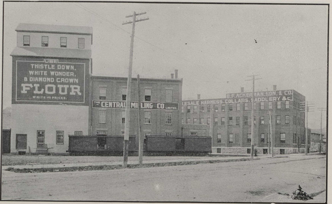
THE CENTRAL MILLING CO., LIMITED—PETERBOROUGH.
