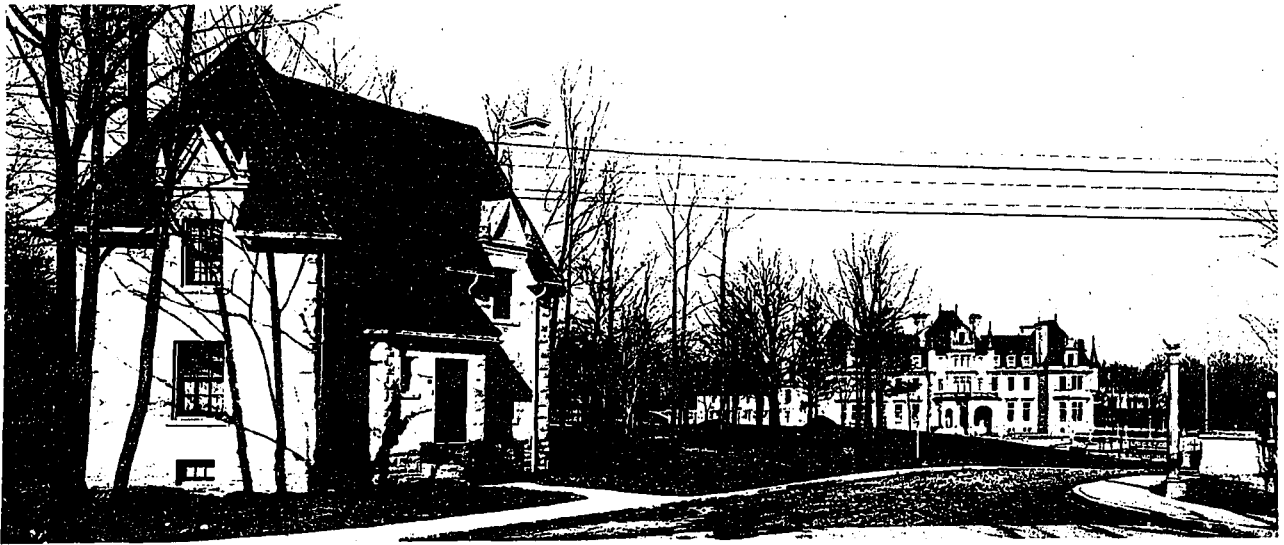
LODGE AND GENERAL VIEW—ONTARIO'S NEW GOVERNMENT HOUSE.
