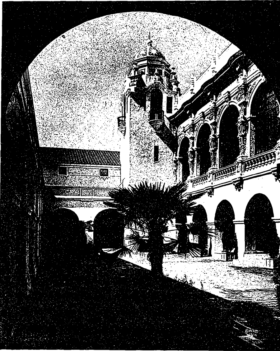
PATIO, SOUTHERN CALIFORNIA COUNTIES BUILDING.
