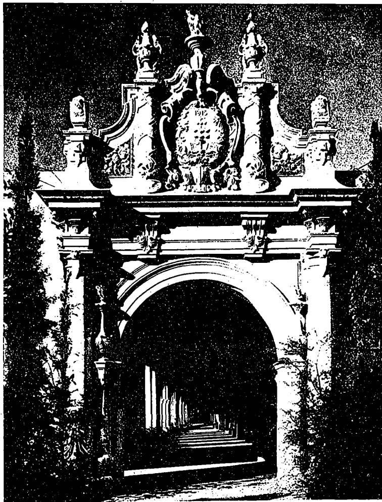
ENTRANCE TO VARIED INDUSTRIES BUILDING.
