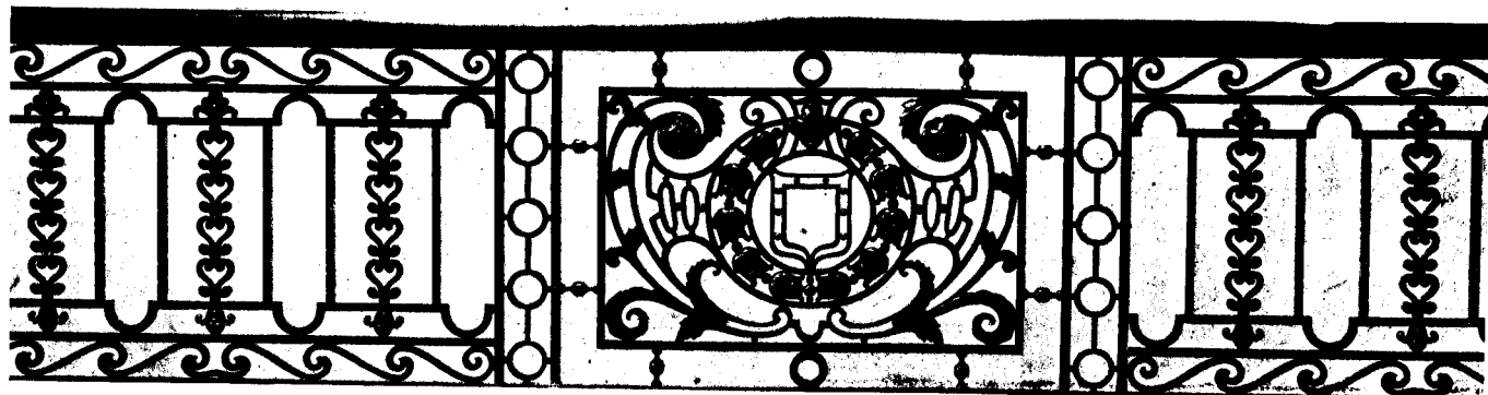
Bronze Railing on Mezzanine Floor overlooking Rotunda.
