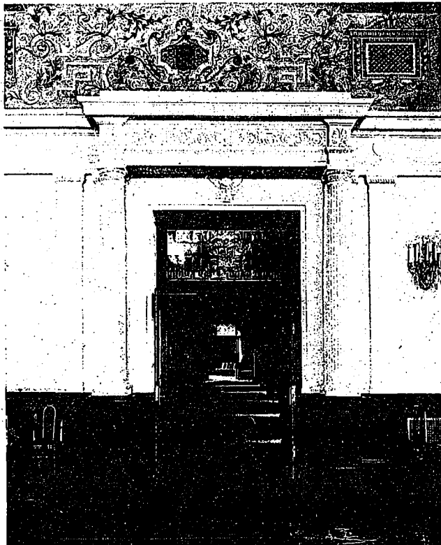
ENTRANCE TO BALL ROOM.
