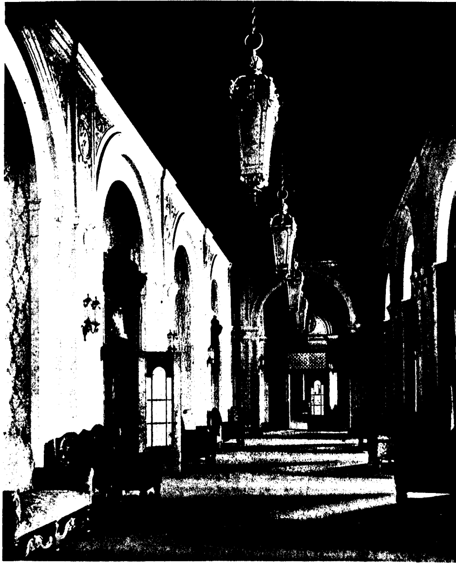
SEVENTH FLOOR LOBBY, FORT GARRY HOTEL, WINNIPEG, MAN. Erected under the direction of Ross and Macdonald, Architects.
