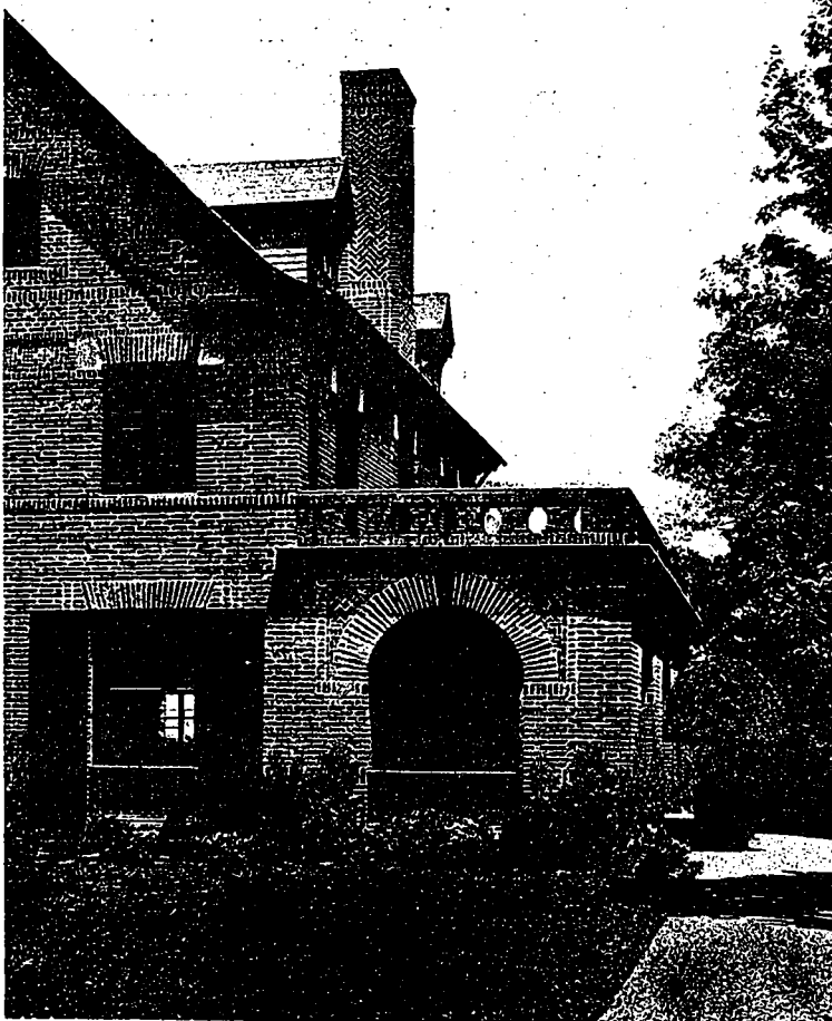
DETAIL OF LOGGIA.
