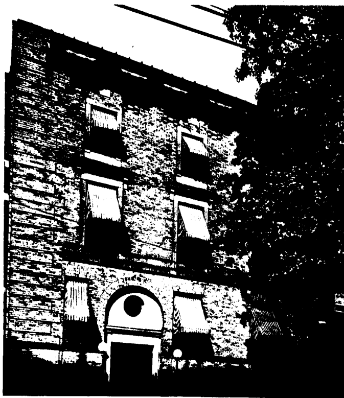
Montefiore Club, Guy Street, Montreal. Saxe & Archibald, 59 Beaver Hall Hill, Architects.
