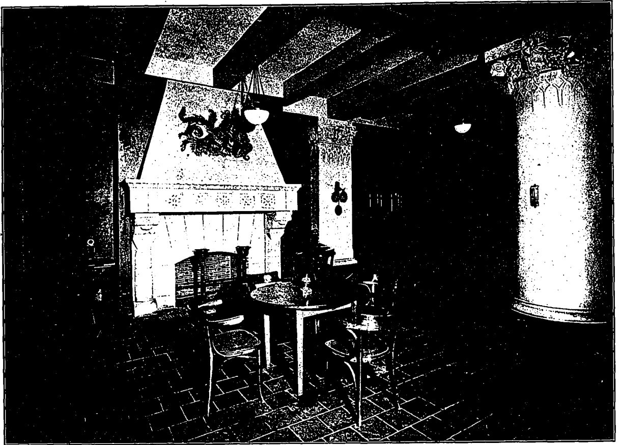
Detail of Mantel in Bar Room, which is of Carved Ohio Stone. E. & W. S. Maxwell, Architects.
