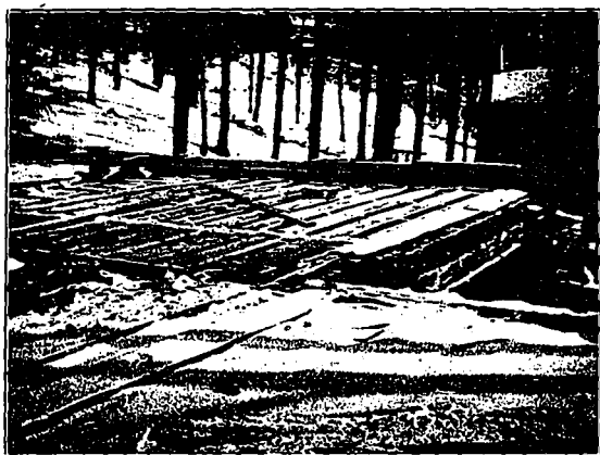
Fig. 8. Upper Form Work for Floors, Consisting of 2 x 10-inch Planks Placed 17 Inches Centre to Centre.
