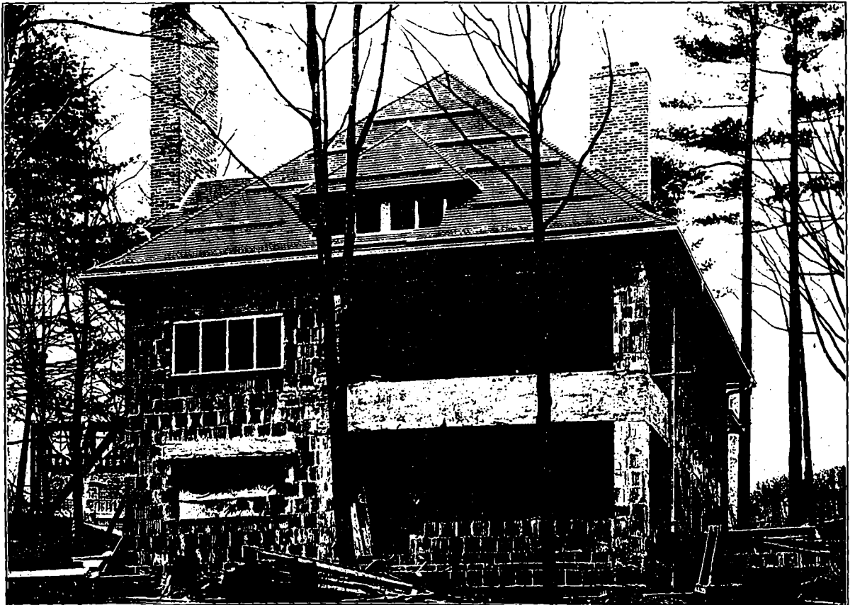
View Showing Wall Construction Before Stucco was Applied.
