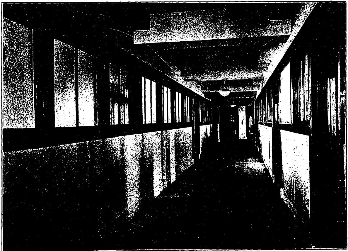
Typical Corridor in White Marble and Mahogany Wood, with Borrowed Lights of Chipped Glass and Grey Tennessee Marble Floor E. & W. S. Maxwell, Architects.
