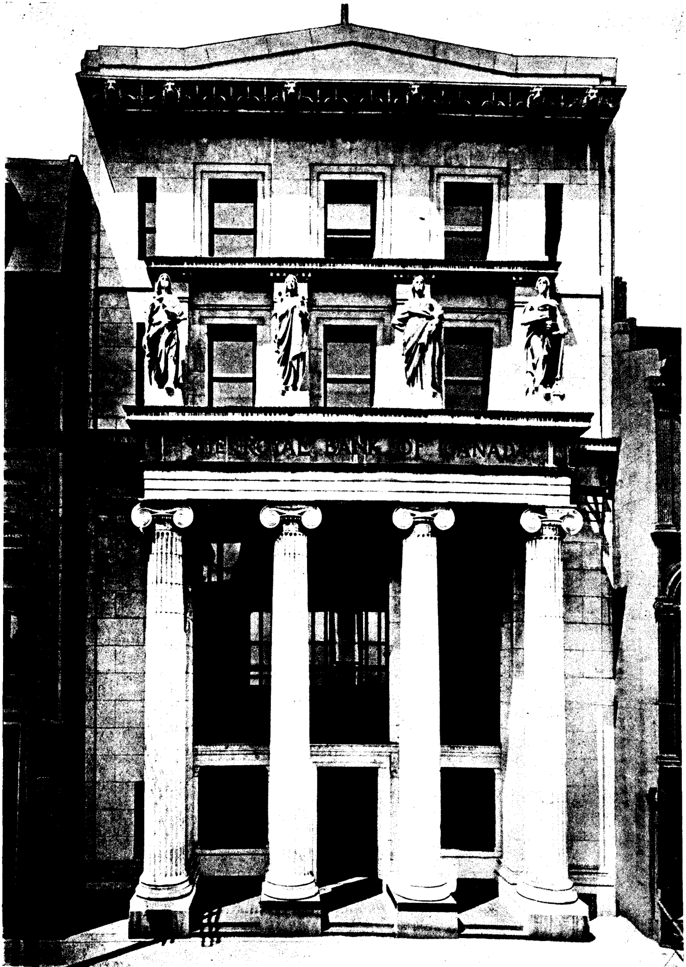
Royal Bank of Canada, St. James Street, Montreal. Howard C. Stone, Architect. Garth & Co., Plumbers. Standard Ideal Ware used.
