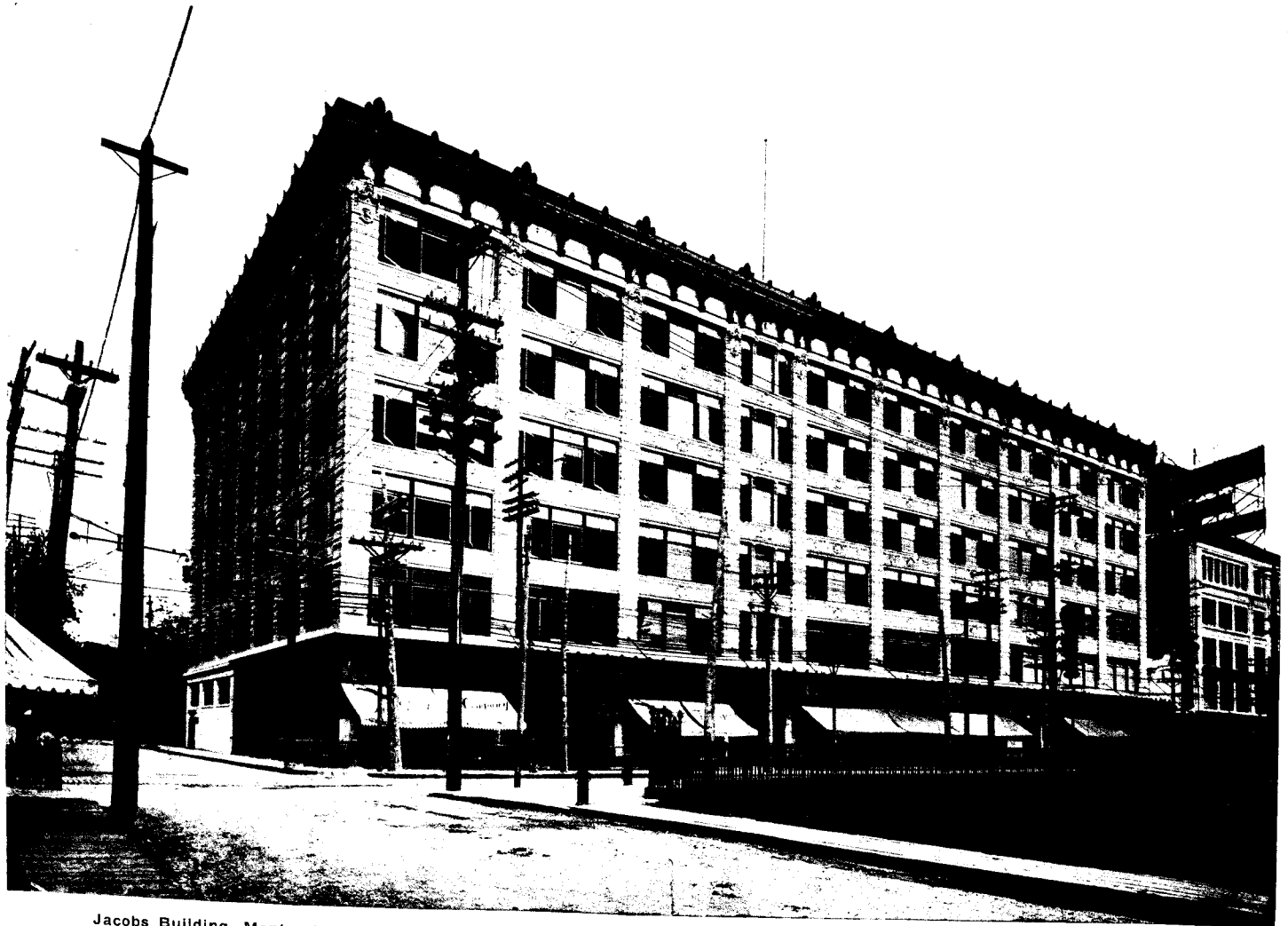
Jacobs Building, Montreal. Mitchell & Creighton, Architects. W. J. McGuire, Ltd., Plumbers. Standard Ideal Ware used.
