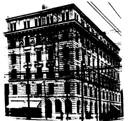
Traders Bank Apartments, Toronto. F. S. Baker, Architect. Don Valley Brick and Porous Terra Cotta Fireproofing used.
