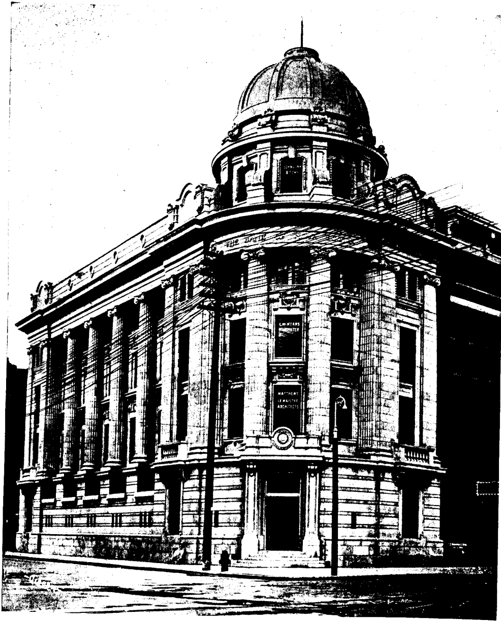
Bank of Nova Scotia, Portage Avenue and Garry Street, Winnipeg. Darling & Pearson, Architects. John Plaxton, Plumber. Fitted throughout with Standard Ideal Ware.
