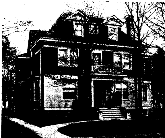
R. H. Metcalfe's Residence, "Norwood," Winnipeg. Wm. Fingland, Architect. Winder & Bowes, Plumbers. Bailey, Starr & Bird, Contractors.
