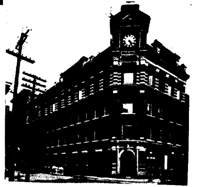
Evening Telegram Building, Toronto. S. J. Curry, Architect. Don Valley Brick and Porous Terra Cotta Fireproofing used.
