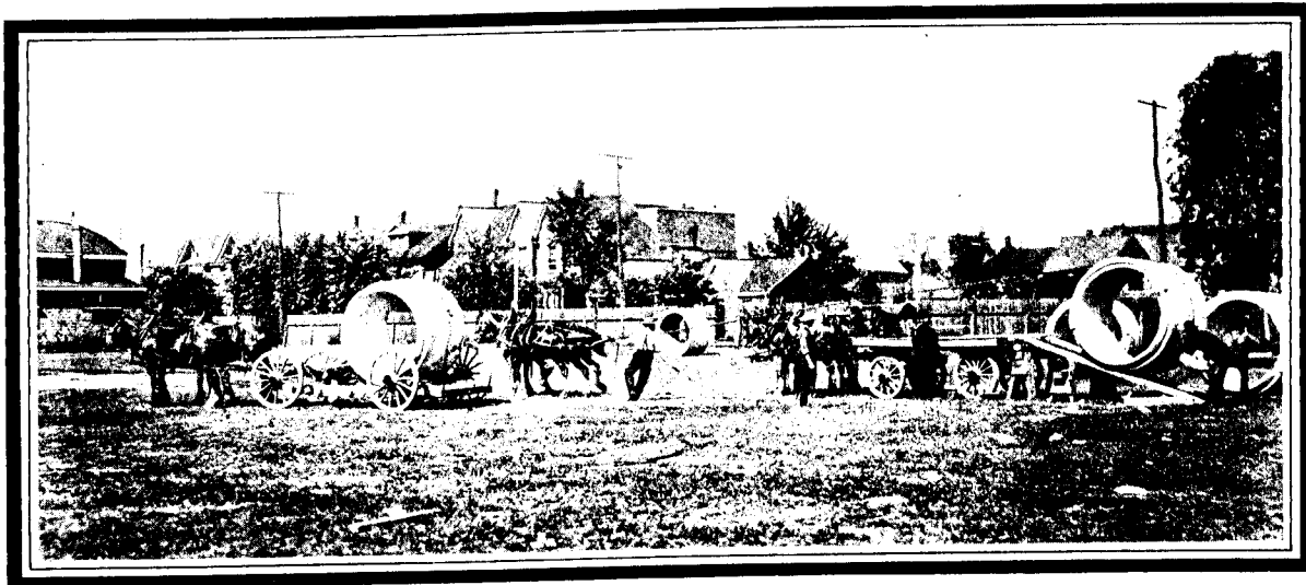
Concrete Pipes for New Trunk Sewer, Toronto. Note the Relative Size of These Pipes, Compared With Men and Horses.
