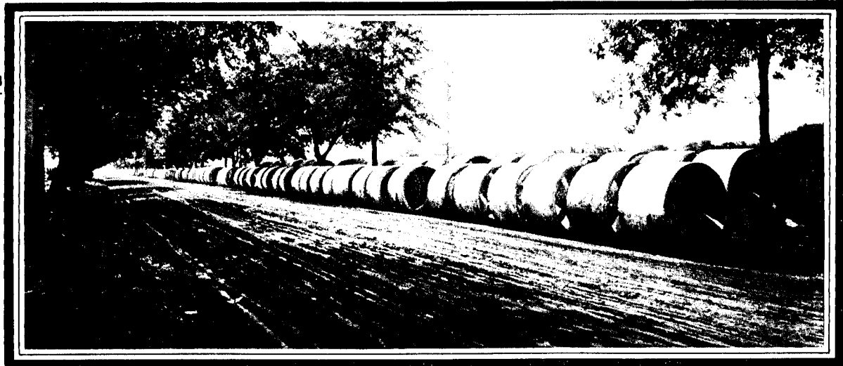
Concrete Pipes for New Trunk Sewer, Toronto. Made by Jennings & Ross, Toronto—under the system of the Reinforced Concrete Pipe Co.
