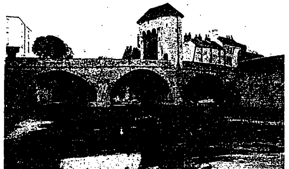
The Monnow Bridge, Monmouth.
