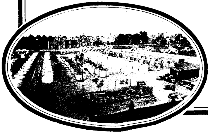
Pipes in Course of Construction.
