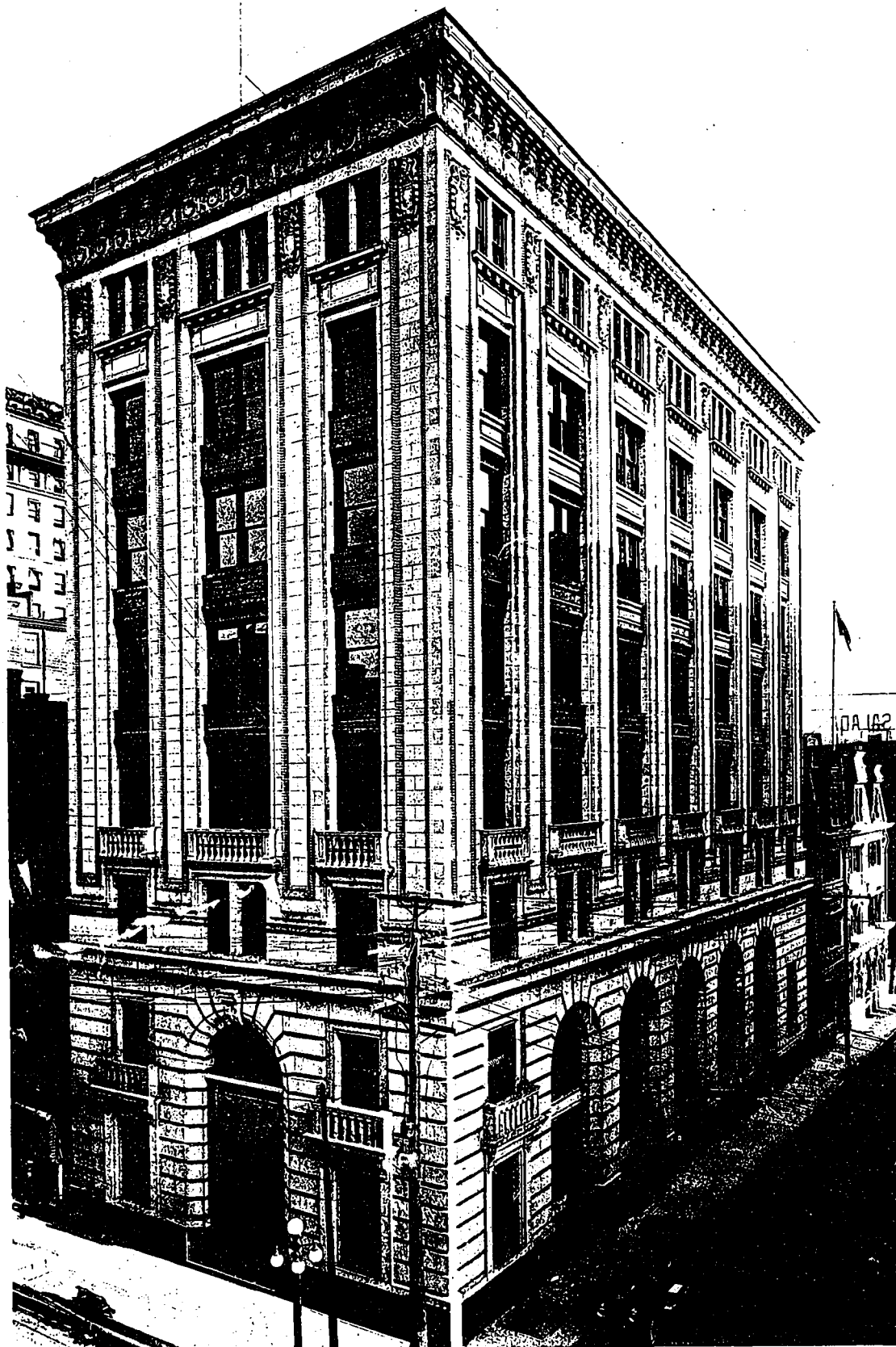
New Premises of the Standard Bank of Canada, South-East Corner of King and Jordan Streets, Toronto. Darling & Pearson, Architects.
