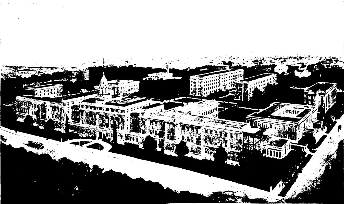
Architects' Perspective, Showing bird's eye view of the Toronto General Hospital, as it will appear when completed. 20,000,000 Don Valley Bricks will be used in these buildings. Don Valley J.A.P. Semi-Vitreous Bricks will be used for all exterior walls. Darling and Pearson, Architects.
