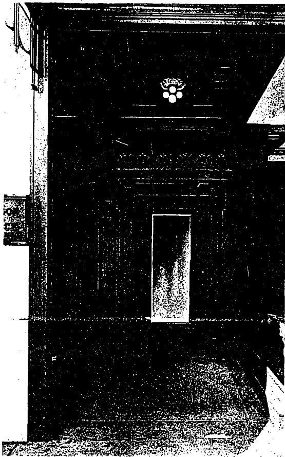
Detail of Entrance, Mason & Risch Building, Toronto. Bond & Smith, Architects.
