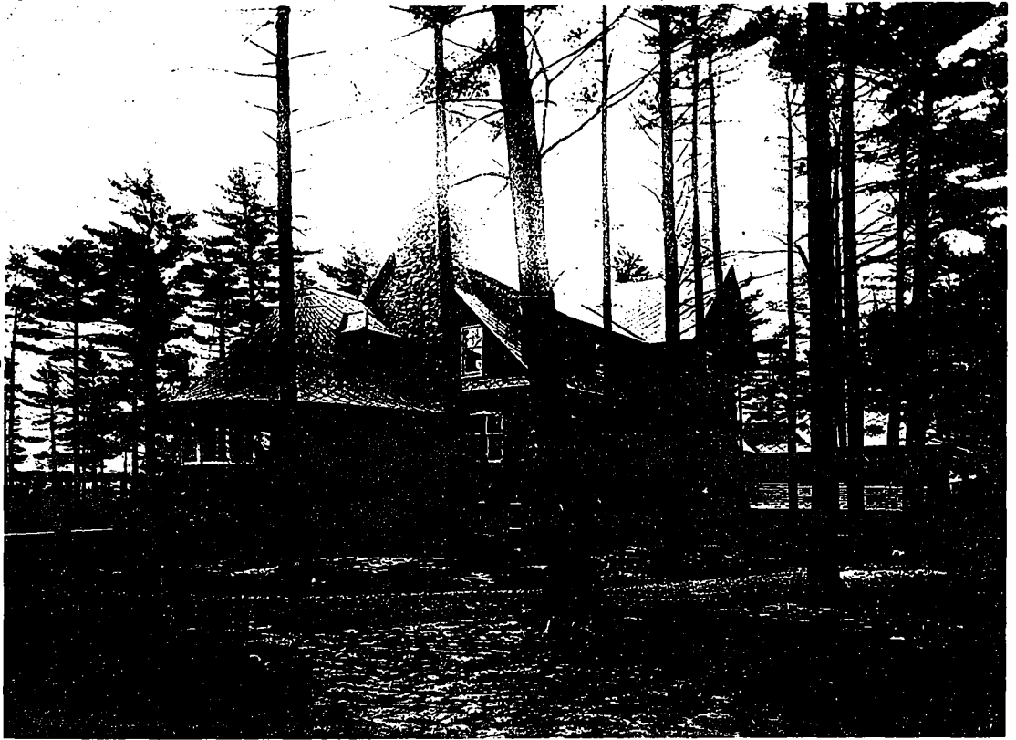
View from North-east.
