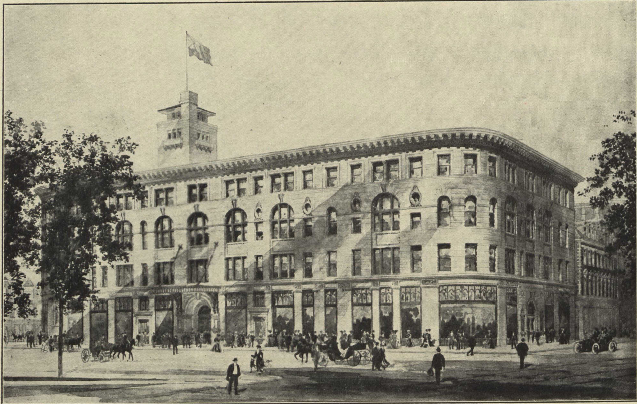
Store of Henry Birks & Sons, Limited, Montreal. Hutchinson, Wood & Miller, Architects.
