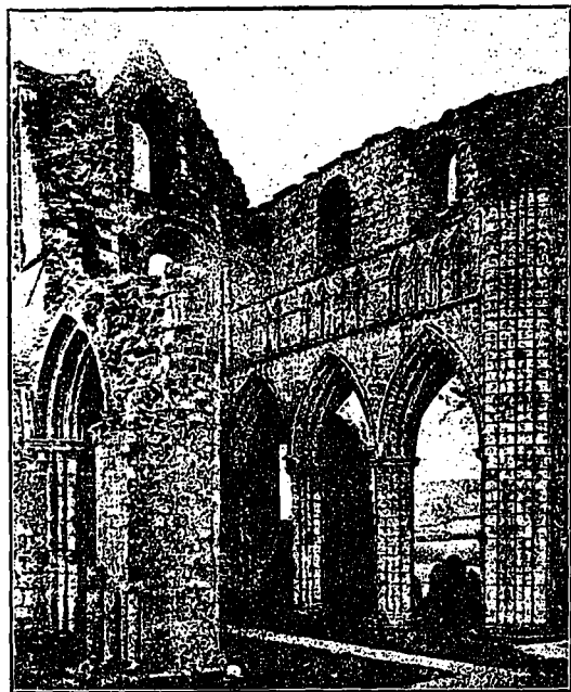
Dundrennan Abbey: North Transept from South Nave Aisle.
