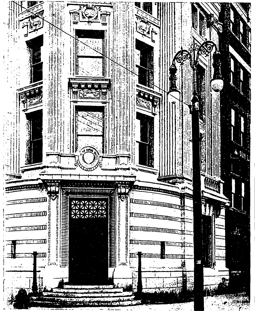
Main Entrance, New Premises, Bank of Nova Scotia, Winnipeg. Showing Detail of Terra Cotta Work. Darling & Pearson, Architects.
