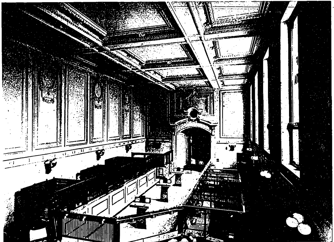
Banking Room, Looking Towards the Entrance, New Premises, Bank of Nova Scotia, Winnipeg. Darling & Pearson, Architects.
