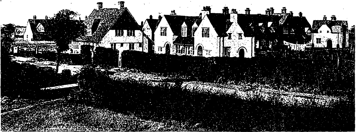
Cottages at Westholm, Letchworth. These Houses were Built by a Co-operative Tenants' Society on a Self Supporting Basis. Note the Extreme Simplicity of the Elevations and Delightful Harmony of the General Scheme. Parker and Unwin, Architects.
