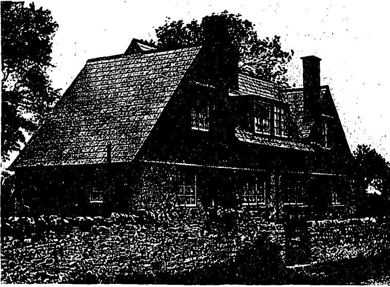
Fair of Cottages at St. Lythans, near Cardiff. These Homelike Little Dwellings Cost $2,400, including the Builder's Profit and the Cost of the Stone Wall in Front. The Walls are of 9-Inch Brick, Roughcasted on the Outside, and the Roof is of Green Slate Carried on Timbers. Speir and Beavan, Architects.
