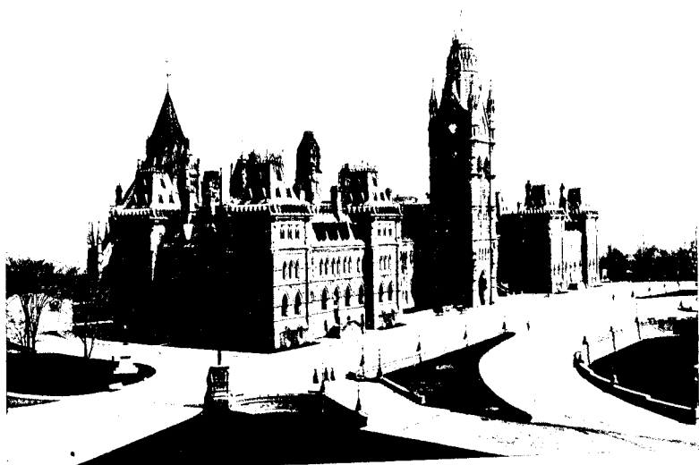
MAIN BUILDING, DOMINION PARLIAMENT, OTTAWA, ONT. Architect—C. Fuller.
