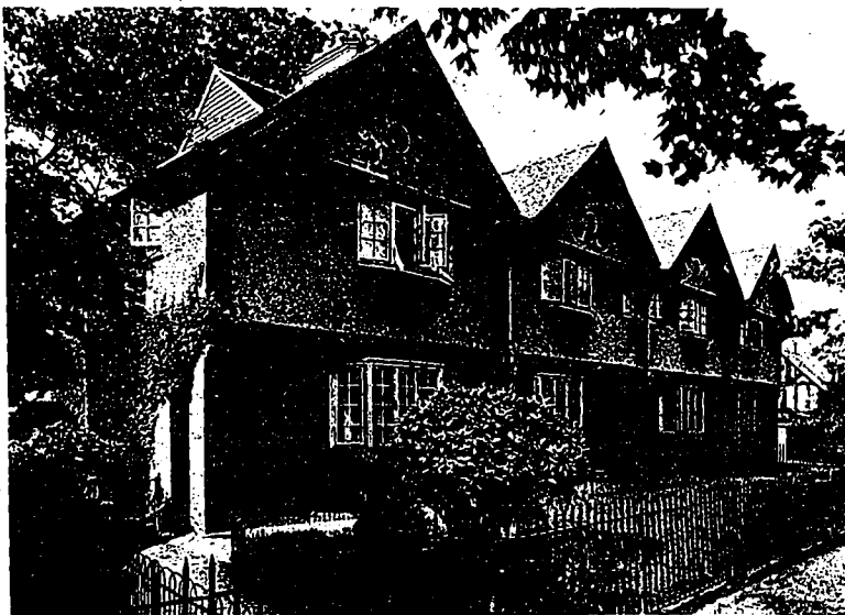
Wood Street, Port Sunlight. In this Row of Cottages the Walls are of Brick, Rough-casted in the Upper Portion and Finished with Decorative Plaster Work in the Gables.
