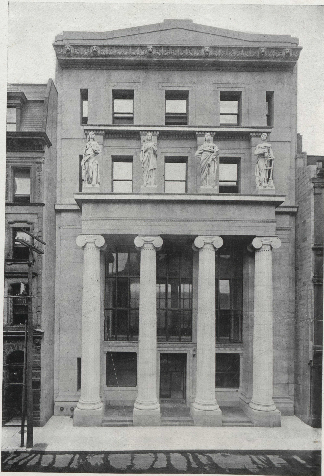
ROYAL BANK BUILDING, ST. JAMES STREET, MONTREAL. HOWARD C. STONE, ARCHITECT. GARTH & Co., PLUMBERS. THIS MAGNIFICENT NEW BANK BUILDING WAS EQUIPPED THROUGHOUT WITH PLUMBING WARE, MANUFACTURED BY THE STANDARD IDEAL COMPANY, PORT HOPE, CANADA.
