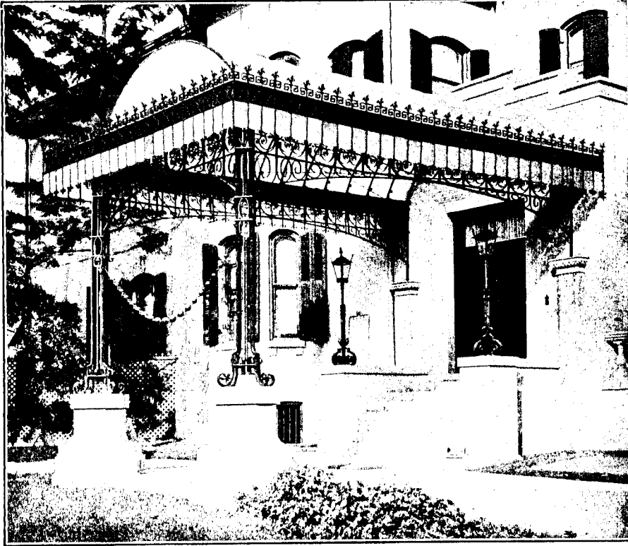
Porte Cochéré, an example of our Ornamental Iron Work.
