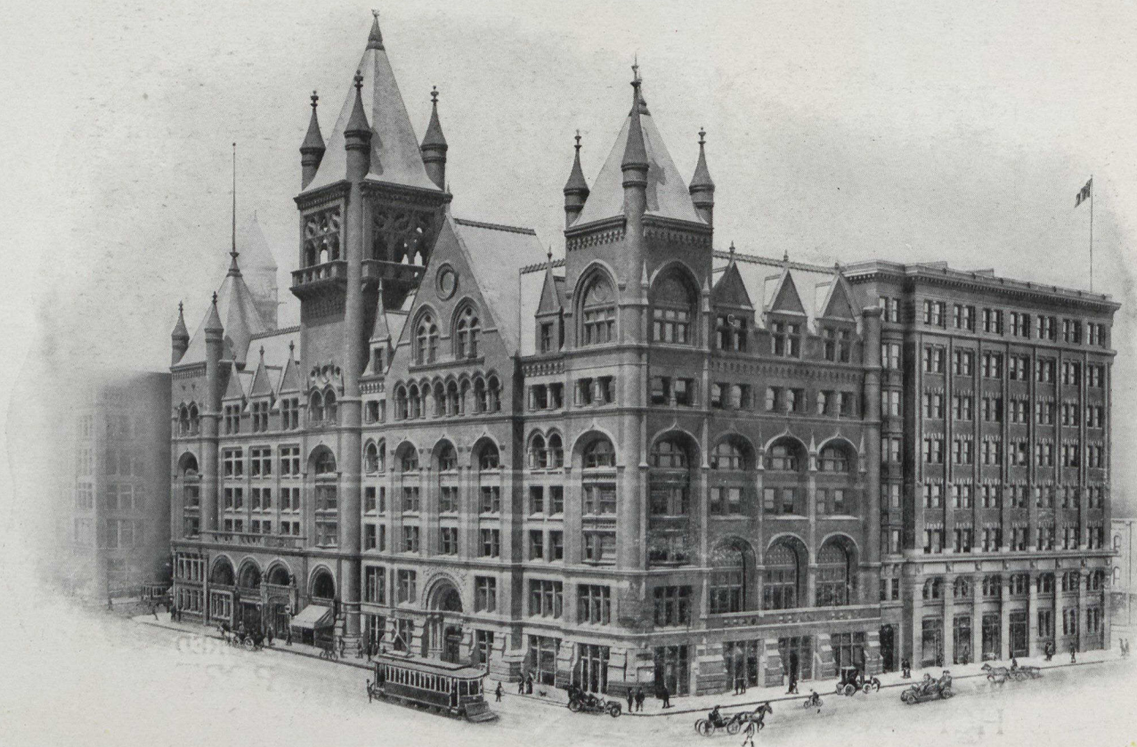
THE CONFEDERATION LIFE BUILDING, TORONTO, SHOWING THE NEW ADDITION RECENTLY COMPLETED. WICKSON & GREGG, ARCHITECTS. KEITH & FITZSIMONS, PLUMBERS. THIS NEW ADDITION TO ONE OF CANADA'S LARGEST OFFICE BUILDINGS IS EQUIPPED THROUGHOUT WITH PLUMBING WARE MANUFACTURED BY THE STANDARD IDEAL COMPANY, PORT HOPE, CANADA.
