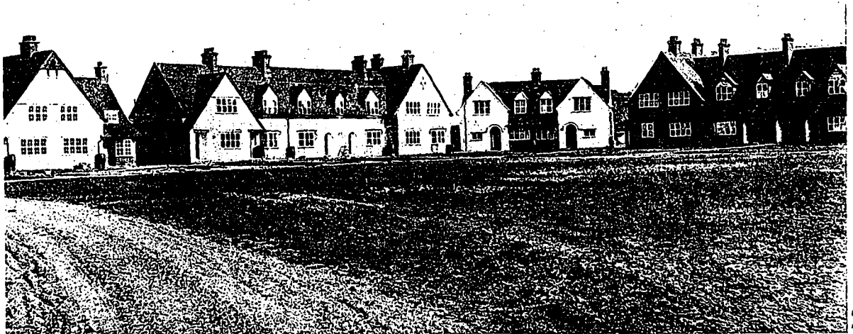
Cottages at Westholm, Letchworth. In Most Cases, the Houses are Built of Brick and Covered with Roughcast Color-washed a Light Cream. The Facing Brickwork is of a Warm Red Color and the Roof is of Hand-made Sand-faced Tile Toned Down to be in Harmony with the Cheerful but Restful Appearance of the Walls.
