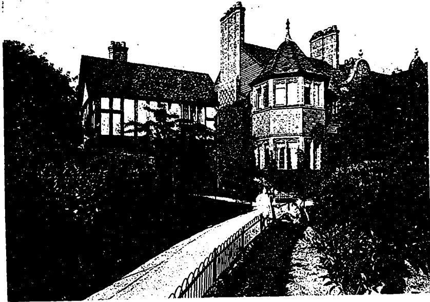
Bridge Street, Corner.
