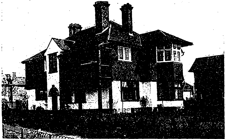
House at Parklangley, Beckenham. One of the Type of Houses Now Being Built According to the Garden Suburb and Town Planning Idea, on a Wooded Estate, About Twelve Miles from London, for Families of the Middle Class. Reginald Fry, Architect.
