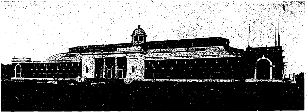
New Transportation Building, Canadian National Exhibition Grounds, Toronto. Built during the past year at a cost of $95,000. In size it is 337 feet long and 153 feet wide. The walls, which are of red pressed brick with Roman stone trimmings, are carried on a solid concrete foundation, while the roof is of the steel truss type, thus making the building practically fireproof. Mr. Geo. W. Gouinlock, Architect.
