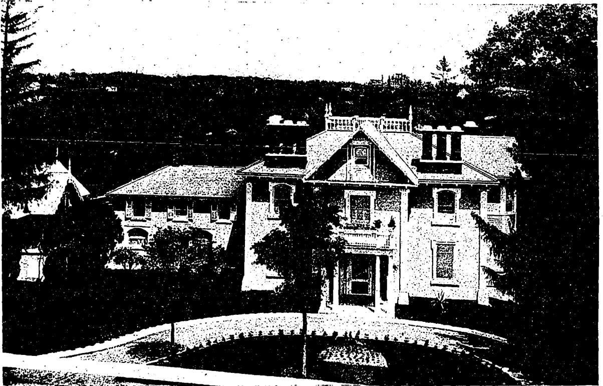
"Inglebush," the Home of Mr. H. T. Bush, Port Hope, Ont., recently remodelled after plans by Mr. J. J. Laferme. This residence, which was built more than fifty years ago for Senator Seymour, is situated on an ideal site, beautifully wooded, and located on an elevation which affords a magnificent view of the surrounding country.
