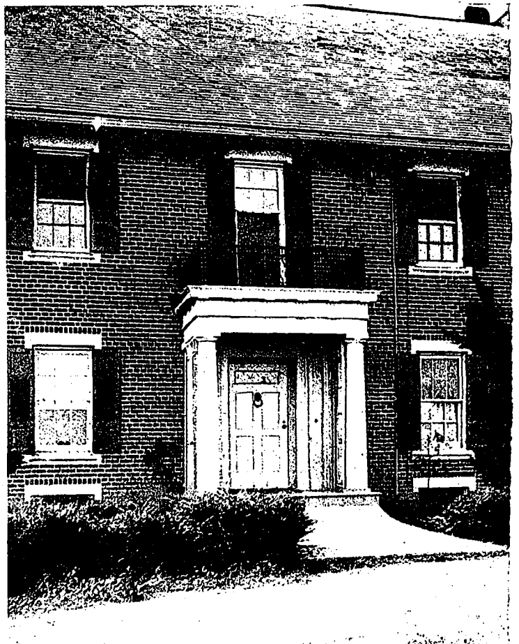
DETAIL OF ENTRANCE.
