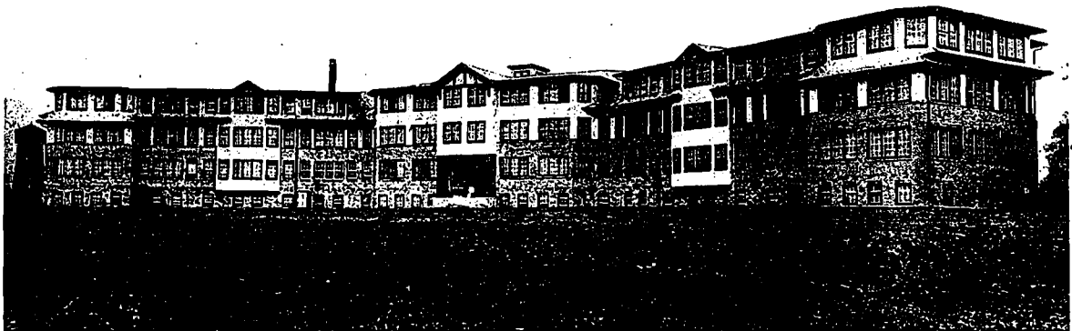
VIEW OF 100-BED INFIRMARY, ERECTED IN CONNECTION WITH TRANQUILLE SANATORIUM, TRANQUILLE, B.C.
