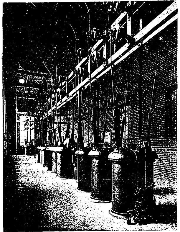
OIL SWITCHES AND BUSES FOR 42,000 VOLT CURRENT.
