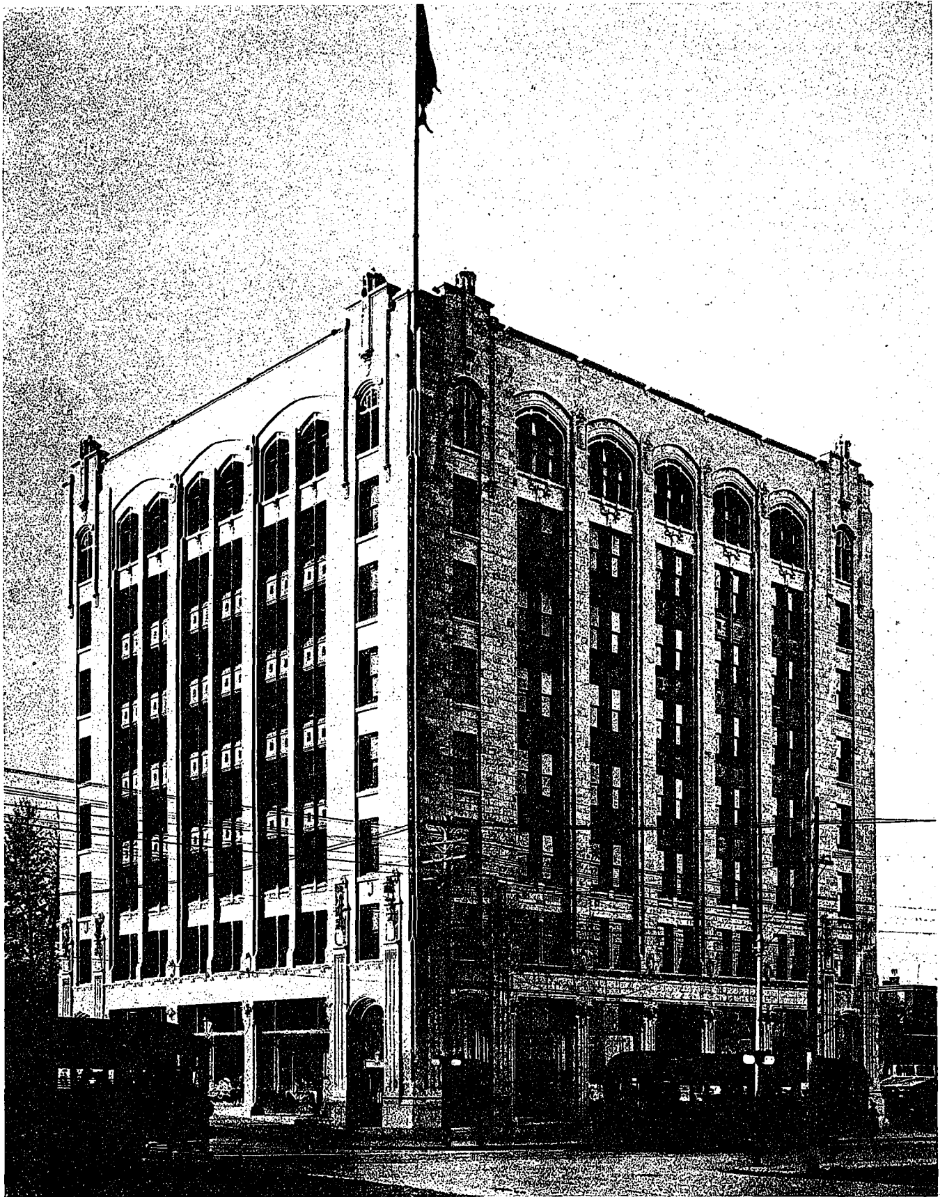
WHALEN BUILDING, PORT ARTHUR, ONTARIO.
