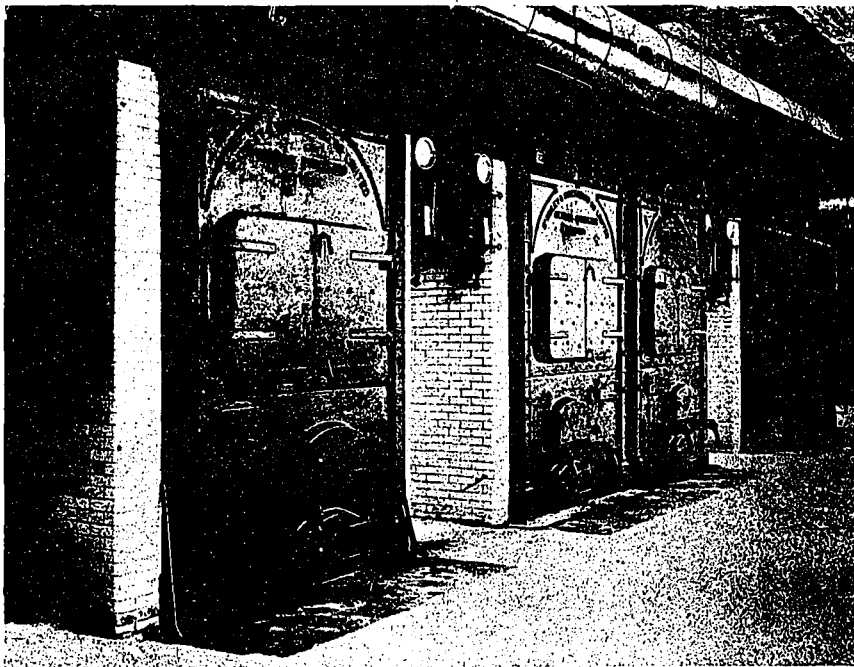
VIEW OF BOILER-ROOM, CUSTOMS EXAMINING WAREHOUSE, OTTAWA.
