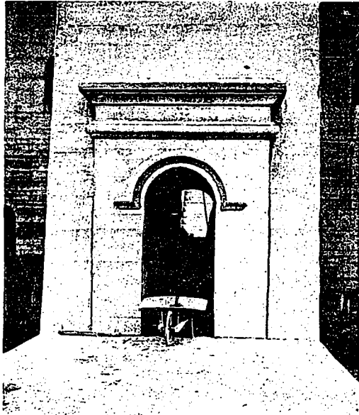
DETAIL OF SMALL CONCRETE PORTAL.
