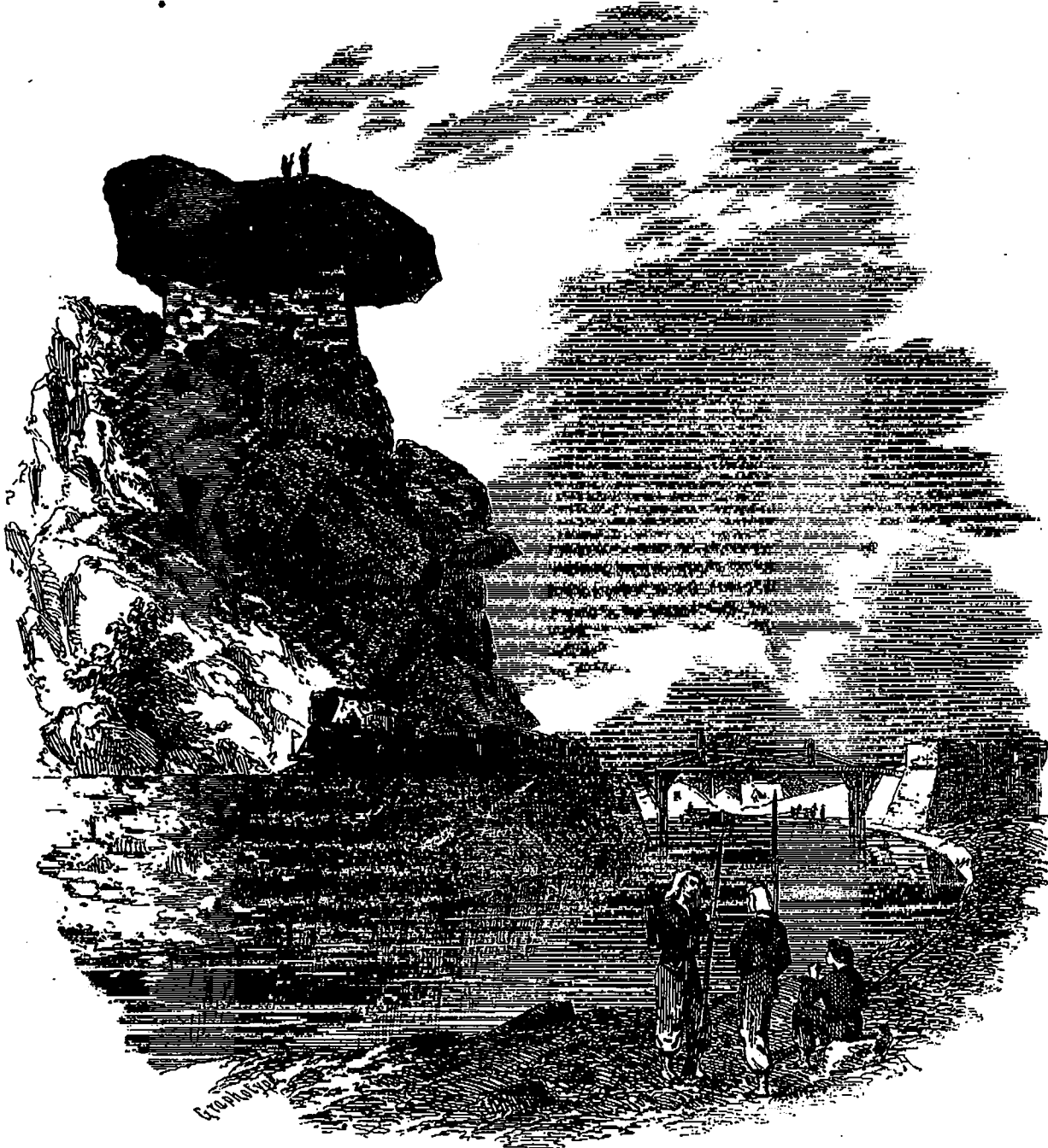
POINT OF ROCKS, NEAR HARPERS FERRY, VIRGINIA.
