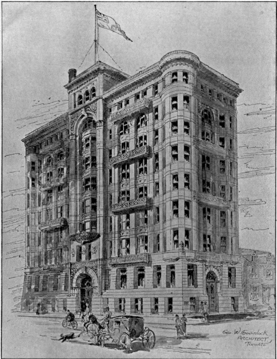
NEW BUILDING FOR THE INDEPENDENT ORDER OF FORESTERS, TORONTO.
