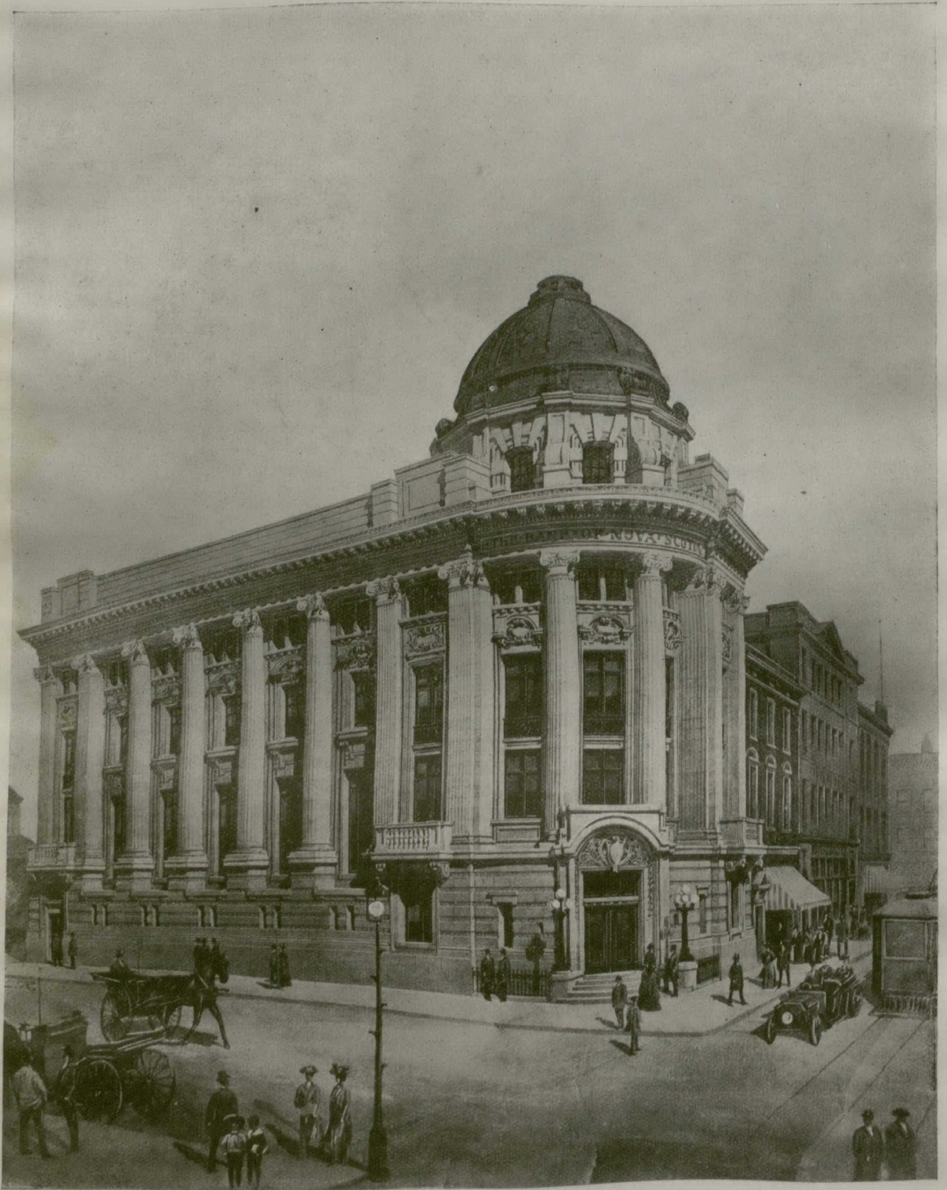
Bank of Nova Scotia's New Winnipeg Building.
