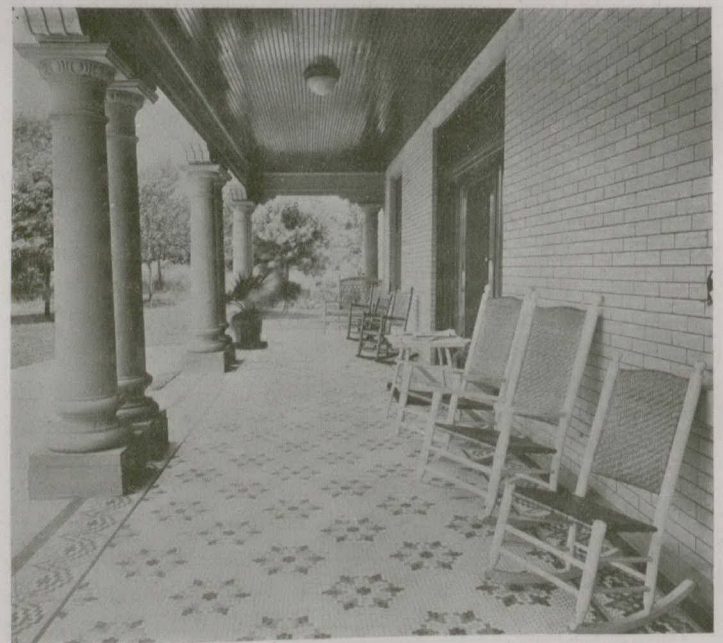
Tiled Porch Floor.
