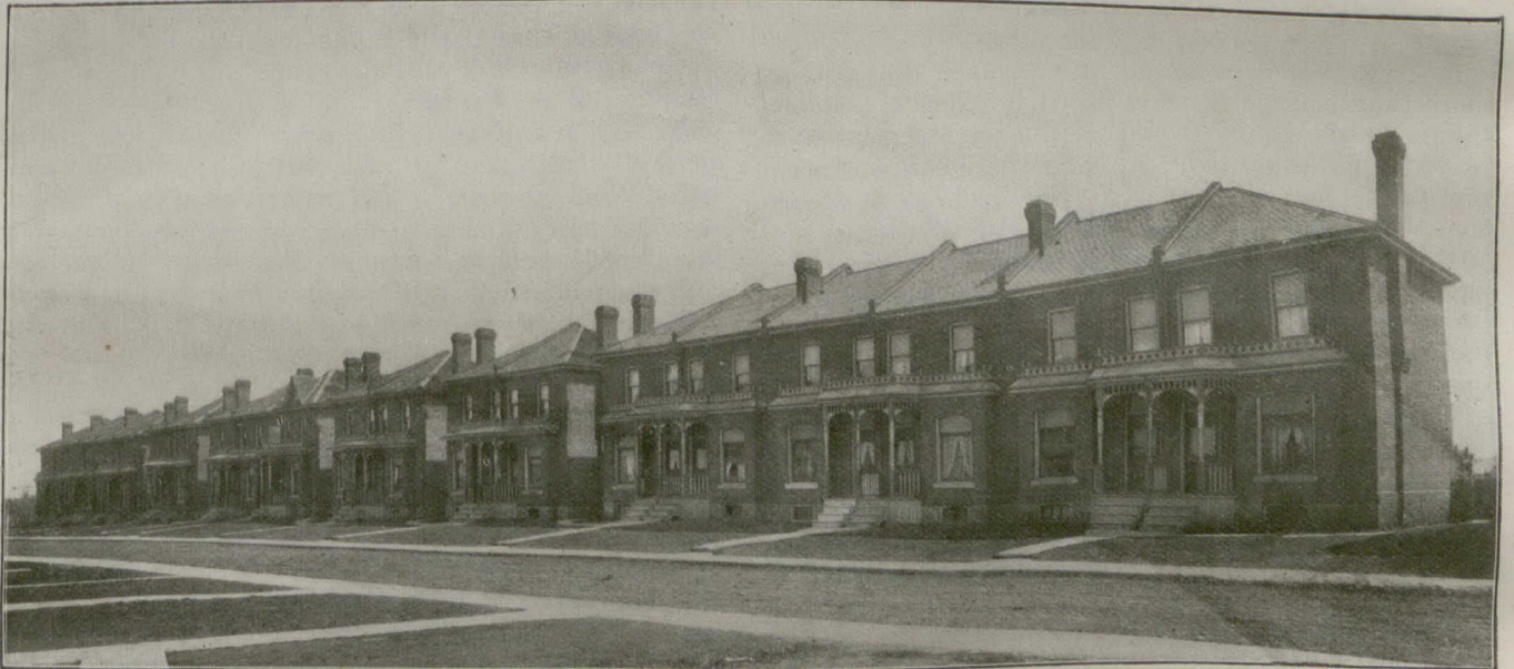
REPRESENTATIVE WORKINGMEN'S HOUSES, EAST FULLERTON AVENUE, HAMILTON, CONSTRUCTED BY THE EASTERN BUILDING SOCIETY (INTERNATIONAL HARVESTER COMPANY.)
